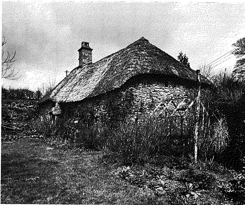
2—HIGHER UPPACOTT, A THATCHED LONGHOUSE AT POUNDSGATE. Longhouses were normally built on a slope, with the cattle housed at the lower end
