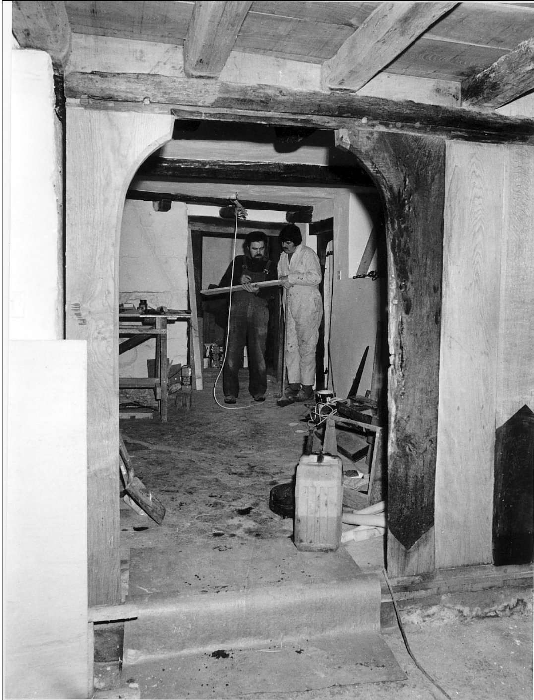
Sanders during restoration.
