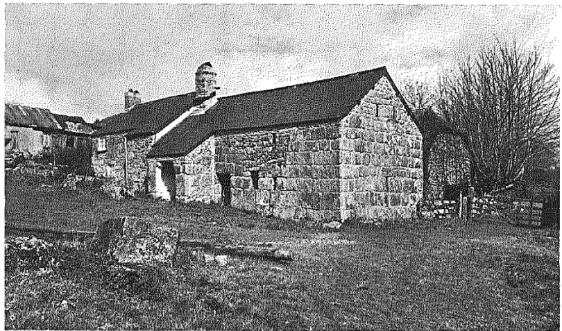
3 and 4—SANDERS, LETTAFFORD, BEFORE AND (below) AFTER RESTORATION BY THE LANDMARK TRUST. "Notable for the size and quality of the ashlar blocks used in much of its construction"
