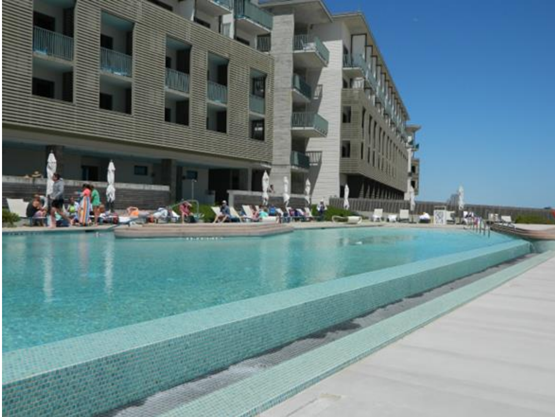
Figure 7. The condensation recovery system at the Lodge provides water for the pool. The system recovers enough water to fill the pool four times yearly (Sasaki, 2018).
