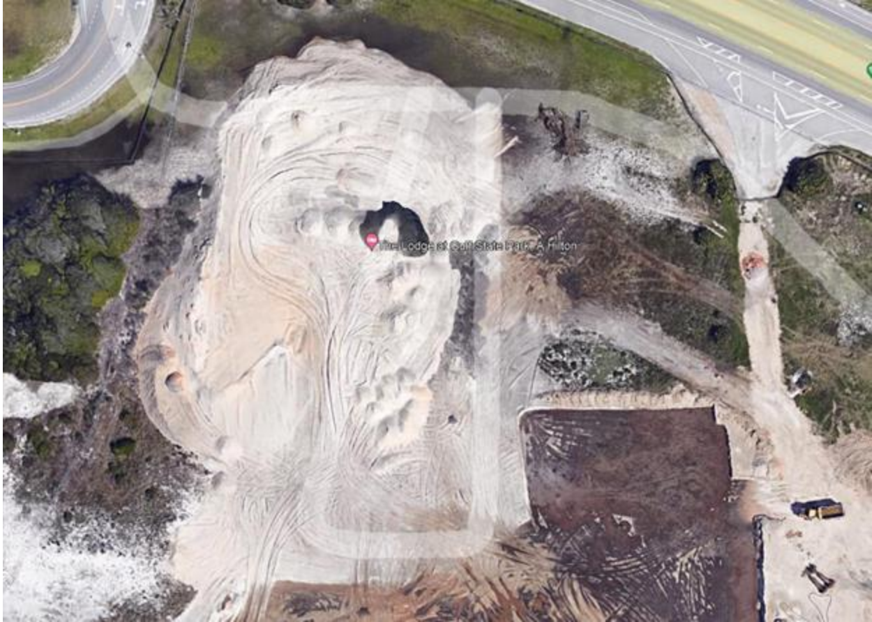
Figure 17. Site of the demolished old lodge at Gulf State Park, Gulf Shores, AL (Google Earth, 1985).
