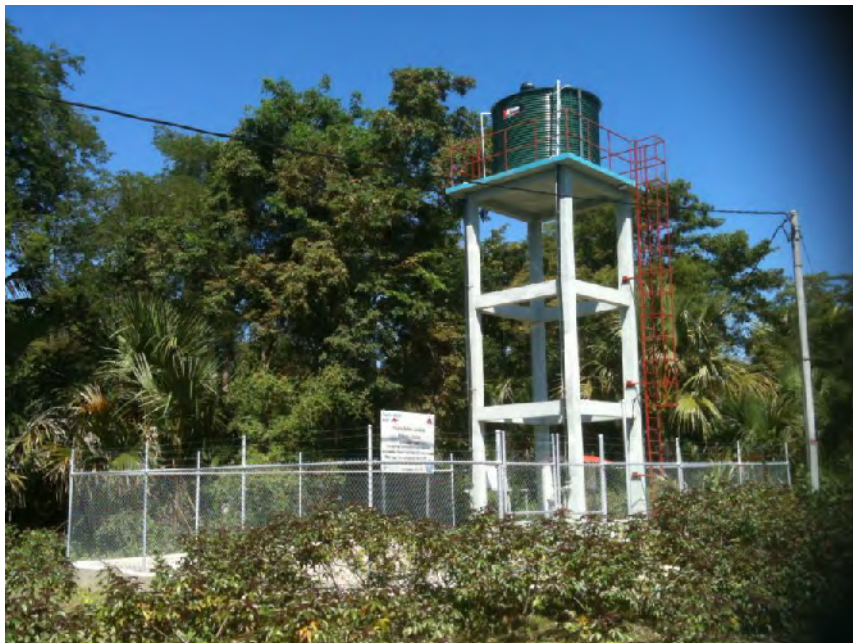
Figure 24 Caravelha Bore at Manulede River
