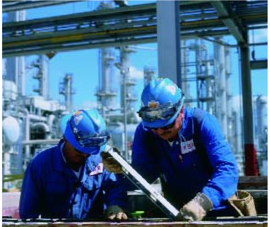
A joint oil and chemicals site, Deer Park, Texas, USA
