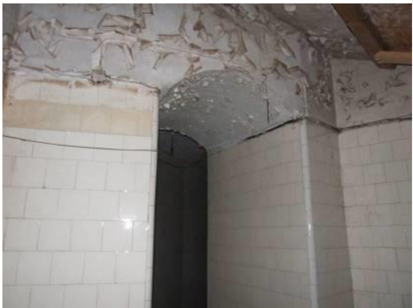
Fabric of the round tower embedded at ground floor
