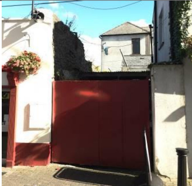
Rubble stone side wall
