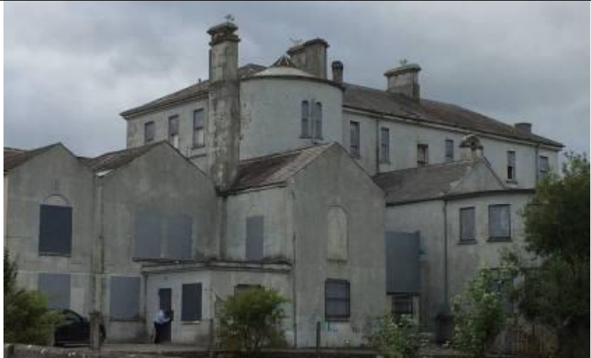
View of rear
