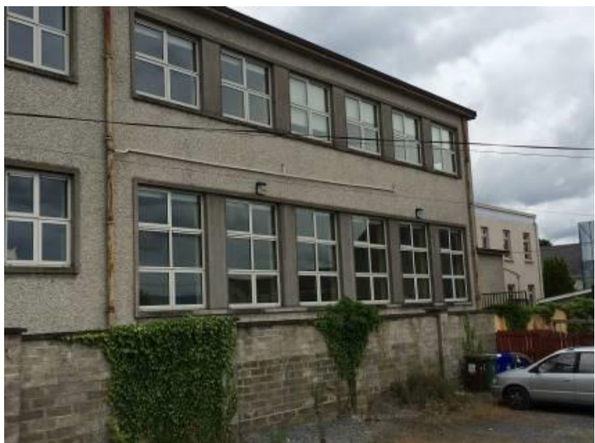
Extension seen from inside the Fort with boundary wall of blockwork
