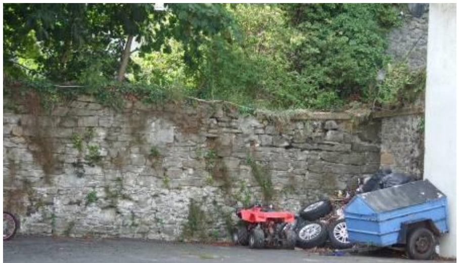
North wall of nave
