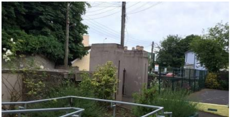
Unrendered inner face of lowered Fort wall on Railway Street
