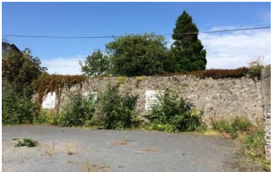
Fort wall forming rear boundary of site
