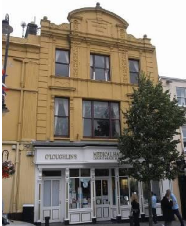
Front elevation of No. 29
