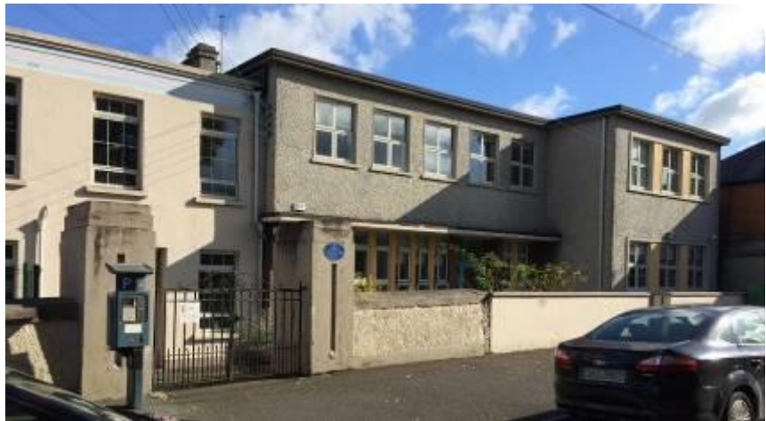
Extension on site of former Pound. Modern boundary retains no fabric of Fort wall
