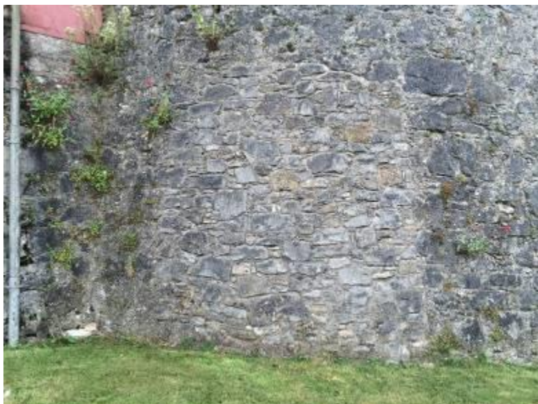
Repaired breach in flanker
