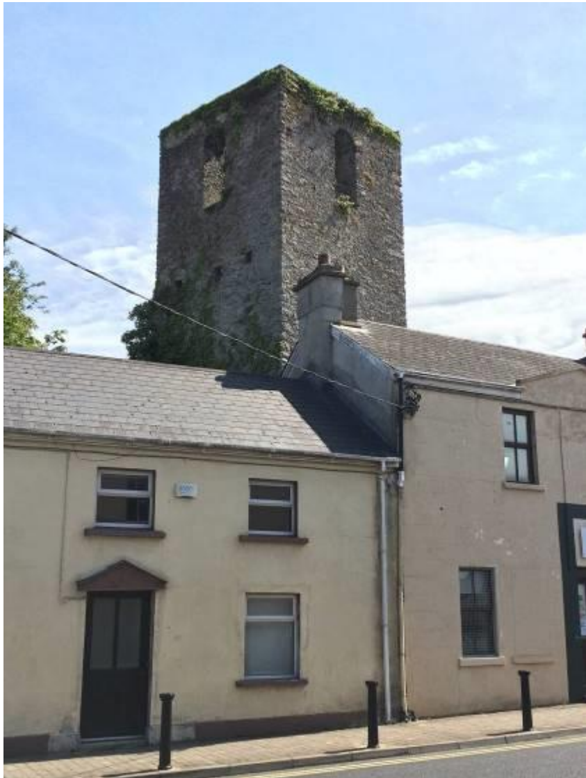
North and west faces of tower seen from Church Street
