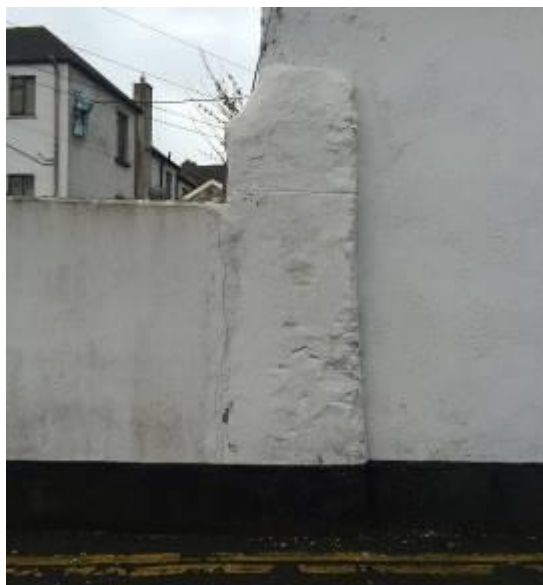
Stub of wall where removed at carpark entrance
