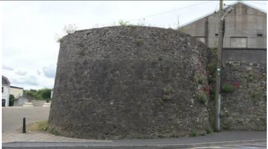
Corner flanker with different masonry in section which rises above walls
