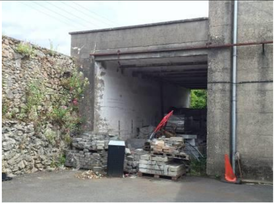
Flat roofed part of industrial building adjoining north wall
