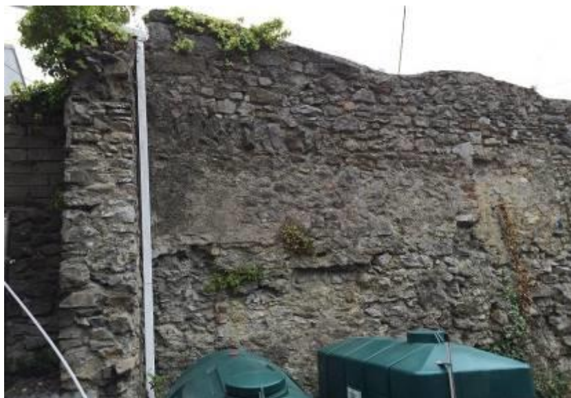
Rubble stone back wall may incorporate fabric of Fort.
