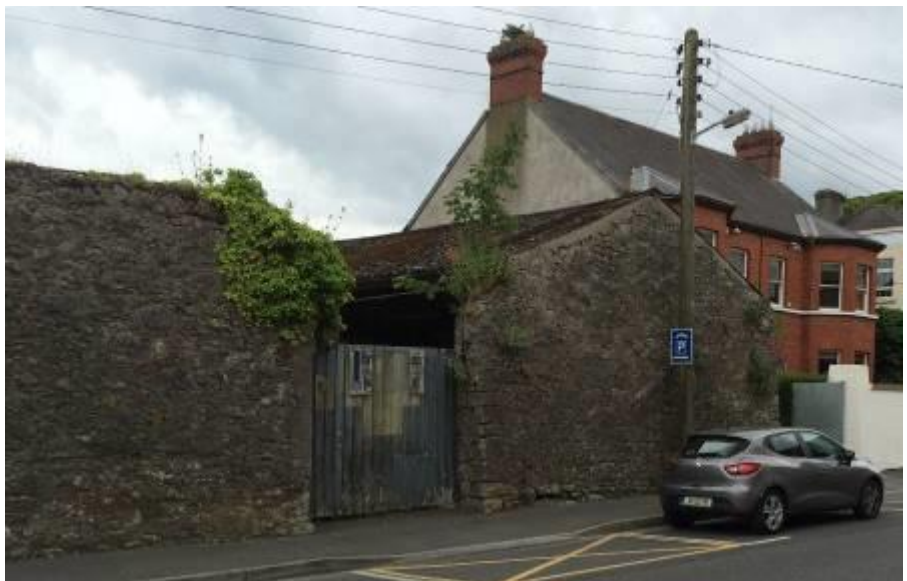
Gateway and battered Fort wall forming gable of western structure
