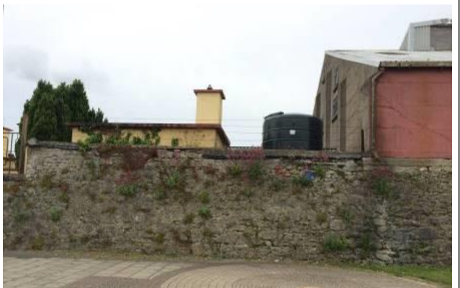
Higher section of wall adjoining mill site
