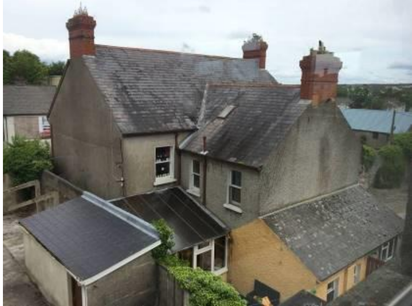
Rear of houses
