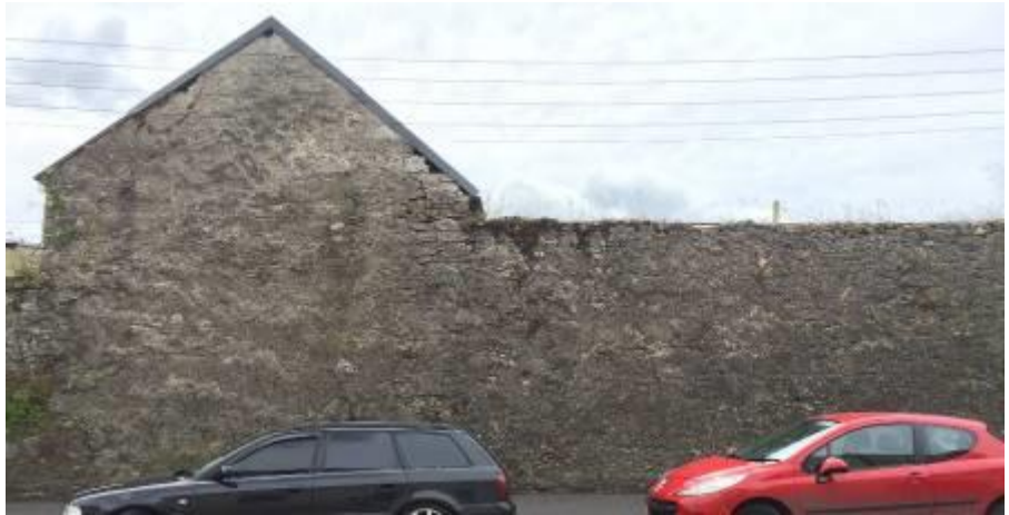
Detail of reconfigured wall
