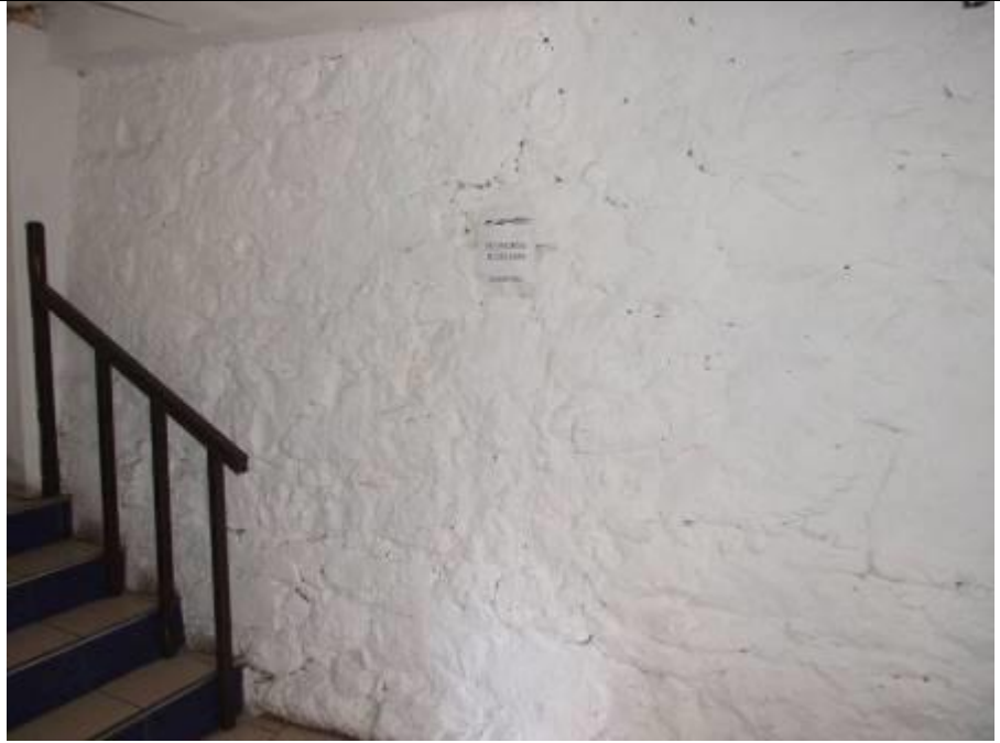
Section of wall to rear of No. 29 within lobby to No. 30
