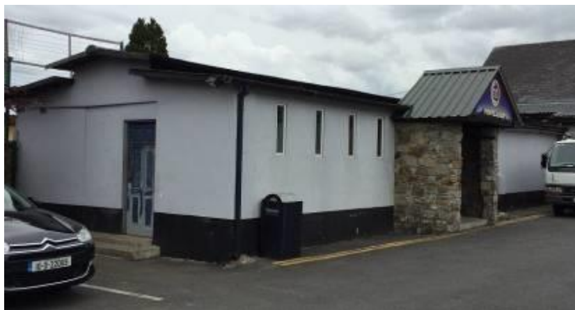
Structure backing onto boundary of Scoil Mhuire (Site 01)
