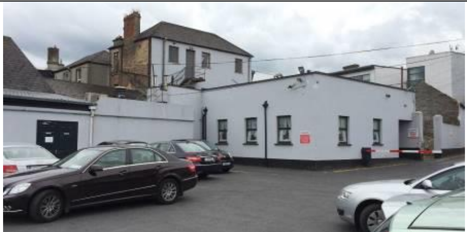
Rear of Hotel. Tall hipped extension lies within the Fort, close to the former Castle.
