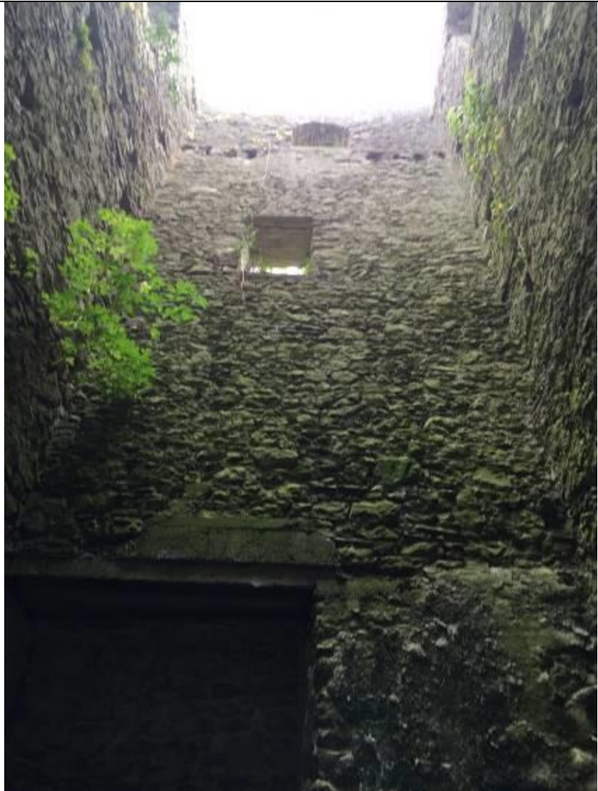
Interior of tower, east side
