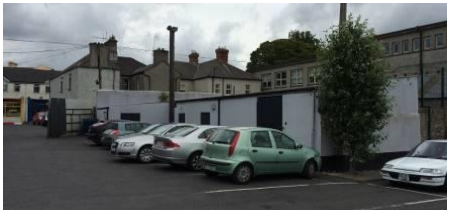
Rear seen from interior of Fort (single storey structure is separate property)
