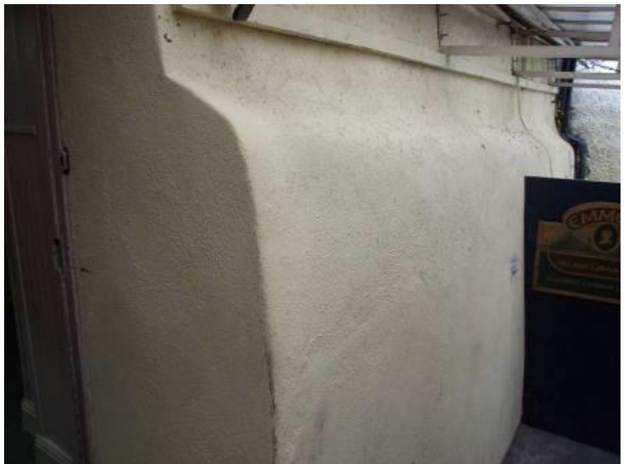
Section of Fort wall in beer garden to rear of No. 29.
