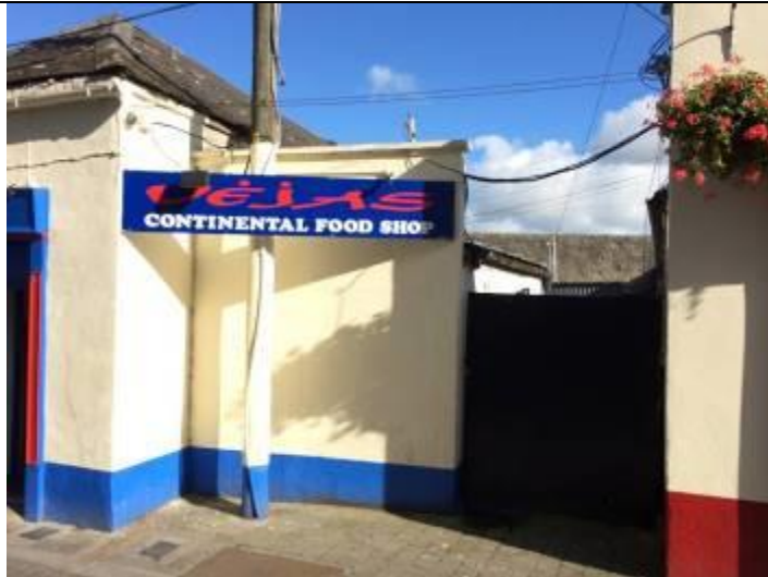
Yard entrance to side
