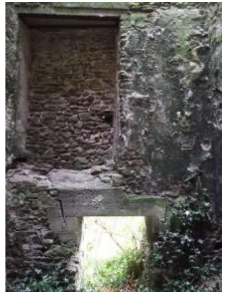
Raised door from tower to nave
