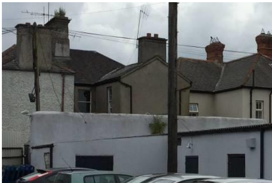
Rear seen from interior of Fort
