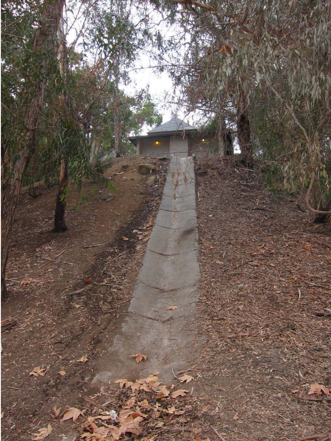
Photo 2: Facing southwest at the drainage located below the restroom building. This drainage appears to be in place to prevent erosion, and to channel water before it sheet flows to the east where it eventually dissipates.
