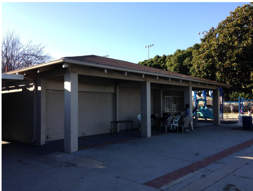
Plate 8. Tennis Shop, view facing northeast
