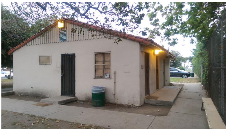
Plate 5. Maintenance building, west and south sides, view facing northeast
