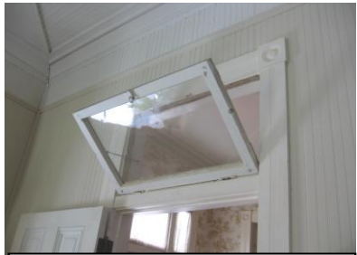
Transom – glassed sash above doors.
