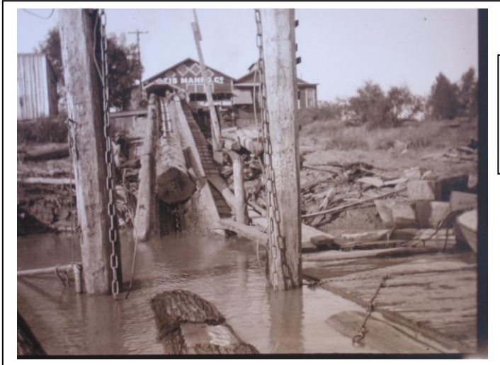
An example of a Jack Ladder, a trough used to pull logs into the mill for sawing into board lumber. Otis House Collection
