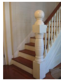
Newel post at bottom of stair.
