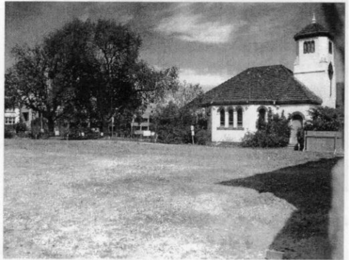
Rear of Chapel with view of carriageway and elm
