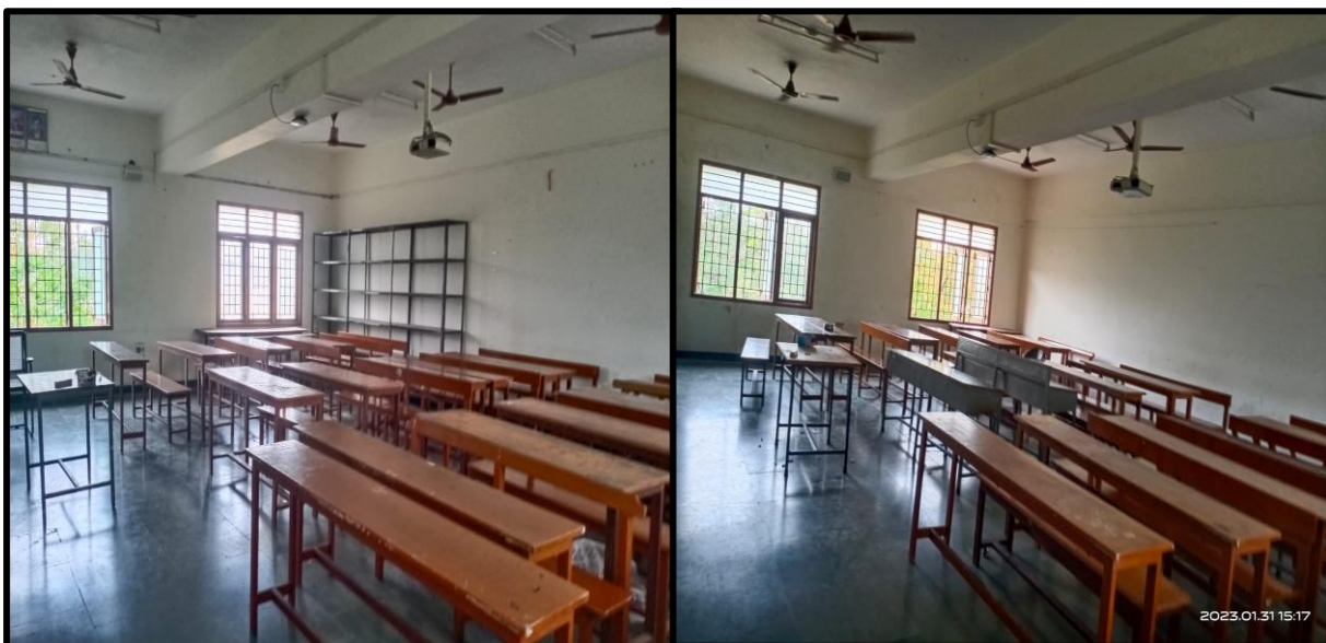
Ventilation Facilities in Loyola College of Education Campus
