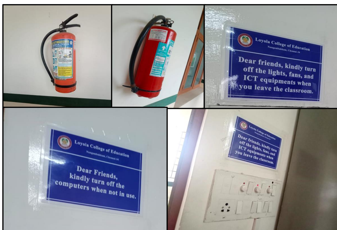
Safety measures and Sign Boards in LCE, Chennai, TN.
