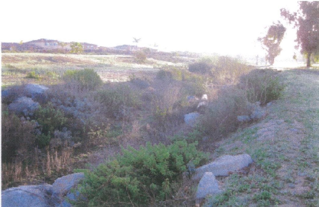
WESTERN BOUNDARY OF DRAINAGE CHANNEL LOOKING EAST
