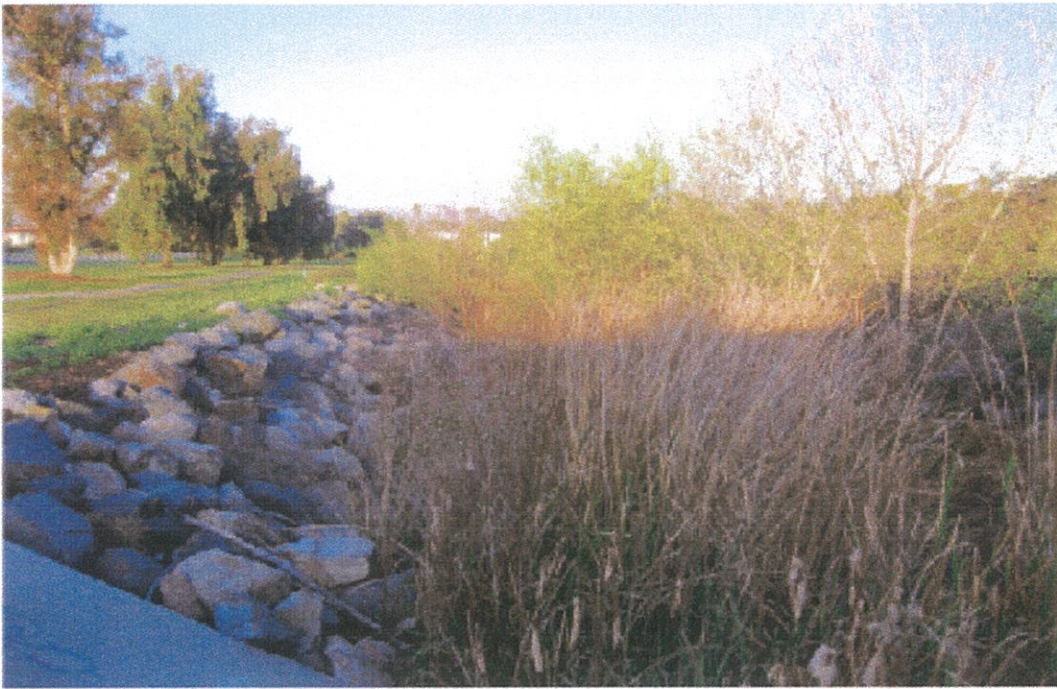
EASTERN BOUNDARY OF DRAINAGE CHANNEL LOOKING WEST
