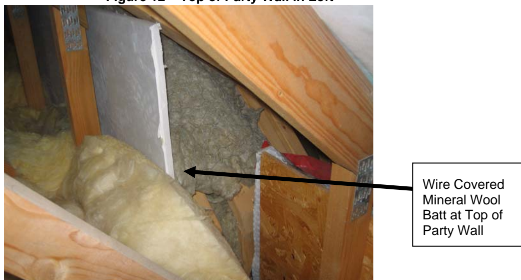
Figure 12 – Top of Party Wall in Loft
