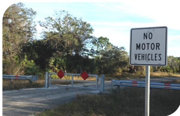
One of the gates installed to deter access by motorized vehicles into HCGCP.
