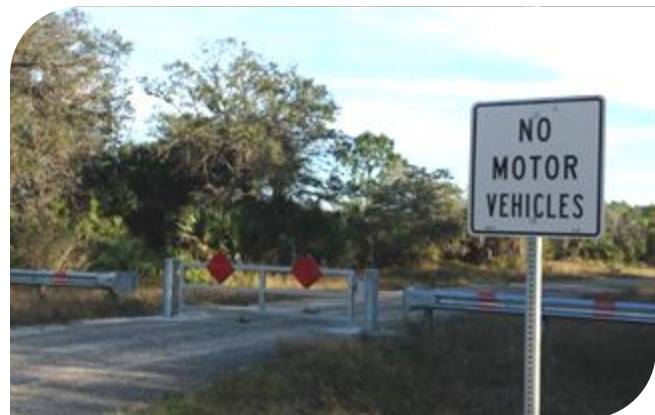
One of the gates installed to deter access by motorized vehicles into HCGCP.
