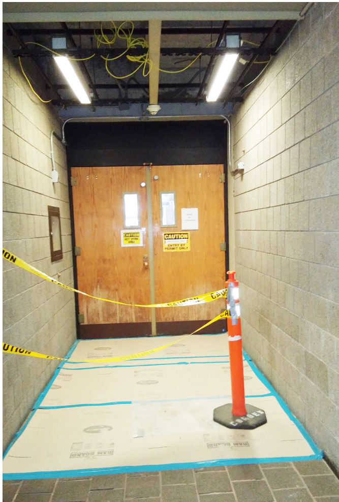
Reconstruction of the Library's first floor in progress
