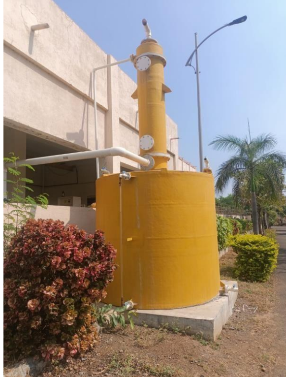
Figure 11: Chlorination unit
