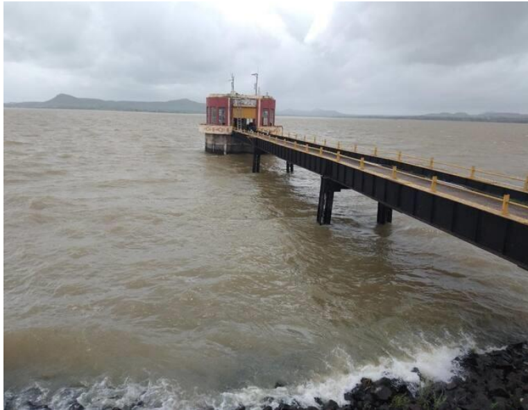
Figure 4: Intake well at Gangapur Dam
