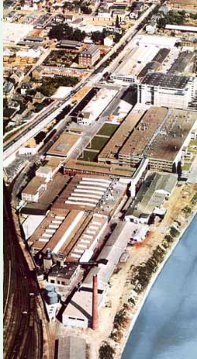
The refrigerated display case plant in Mainz-Kostheim in the 1960s.
