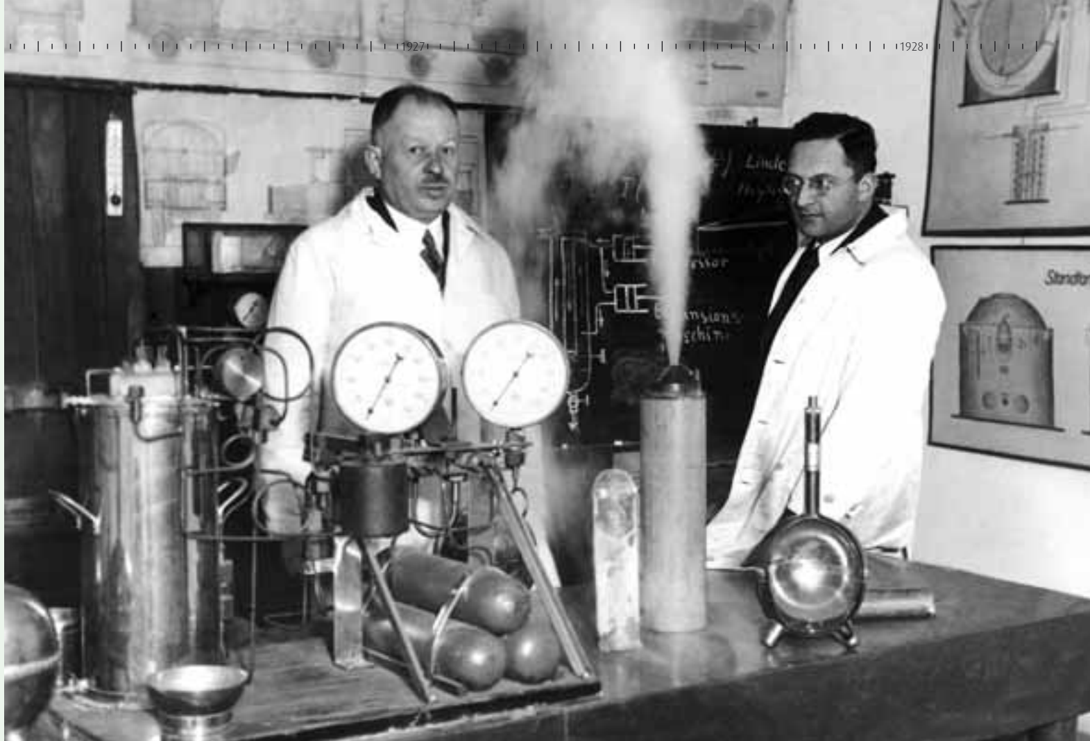
Paulus Heylandt (left) in his Berlin laboratory, approx. 1935. In front on the right is a cutaway model of the transport tank for liquid air, which he developed.
