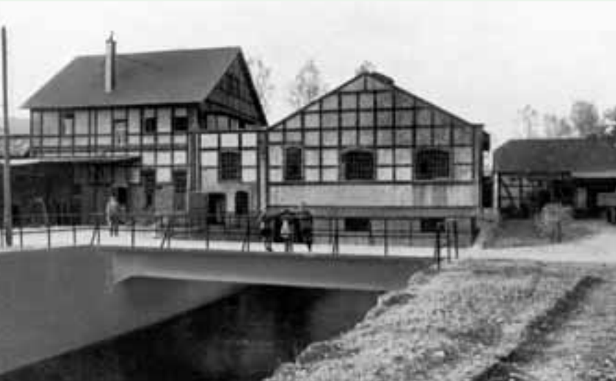
Untermaubach oxygen plant (west of Cologne, approx. 1920).
