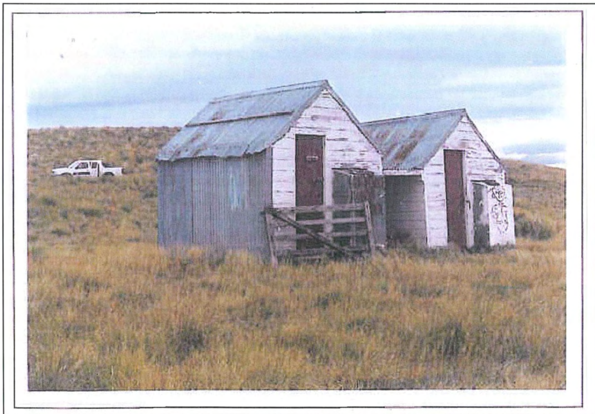
Photo 6. Huts on the Onslow Block
