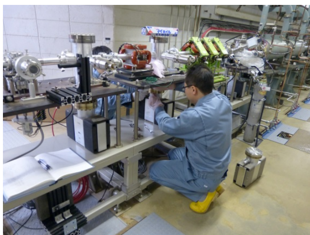
Fig.4. Work for ion pumps replacement.
