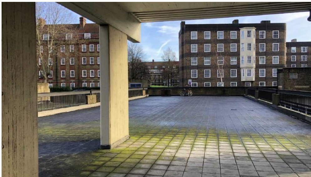
Figure 25: View of terrace at Coverley Point (source Design and Access Statement)
