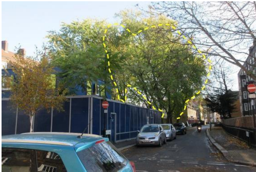
Figure 53: Extract from Tree Report with view looking east on Orsett Street (Yellow line indicates extent of retained canopy)
