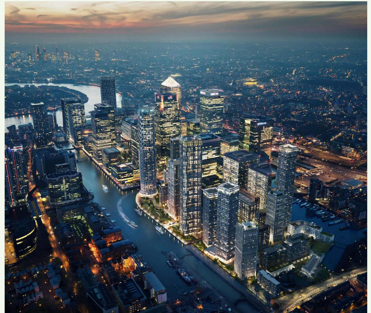
Photographs copyright © canarywharf
