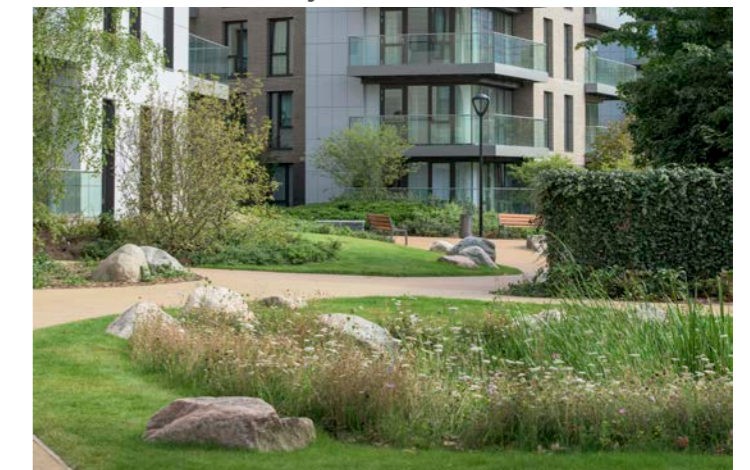
SuDS basin Woodberry Down
