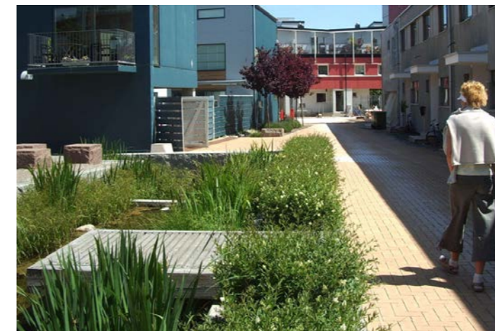
Rain Garden, Malmö Western Harbour
