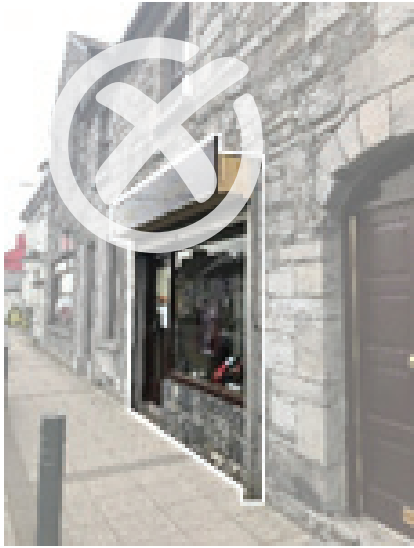
Fig. 25. Projecting roller shutter boxes will not be permitted.
