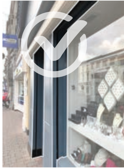
Fig. 27. Roller shutter guides should be integrated into the shop front in rare cases where externally installed roller shutters are permitted.
