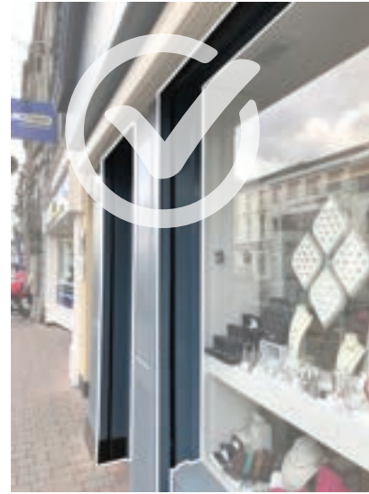
Fig. 27. Roller shutter guides should be integrated into the shop front in rare cases where externally installed roller shutters are permitted.
