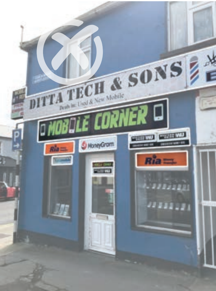
Fig. 12. Excessive signage with double fascia.
