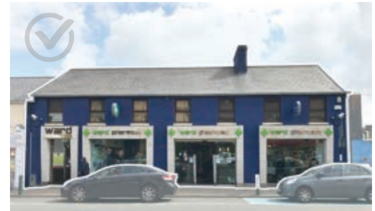
Fig. 4. Quality materials and finishes, and design and proportion respectful of upper floor window locations.
