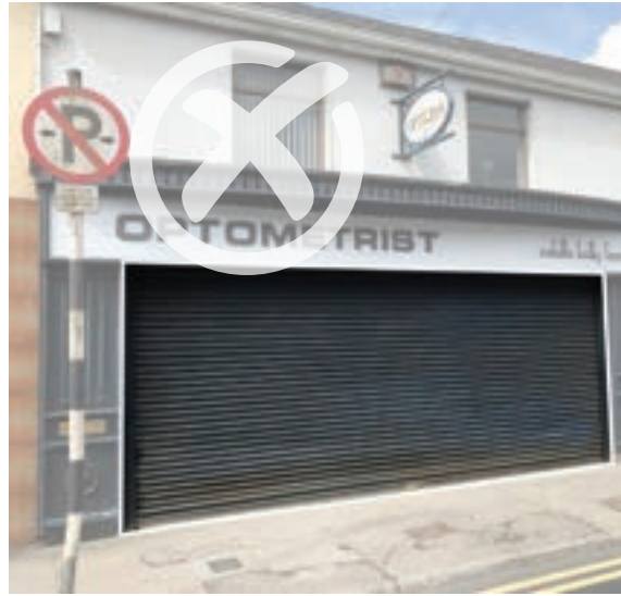
Fig. 26. Externally installed, solid roller shutters will not be permitted.
