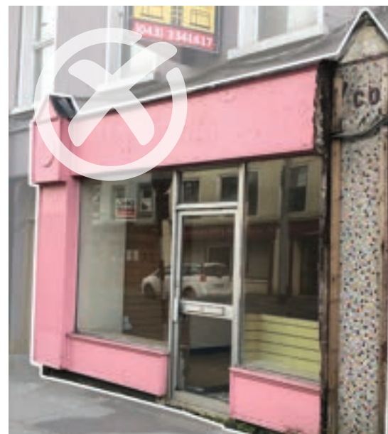
Fig. 20. Lurid colour timber shopfront over decorate original.
