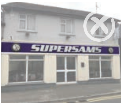
Fig. 32. Overtly large lettering relative to fascia.
