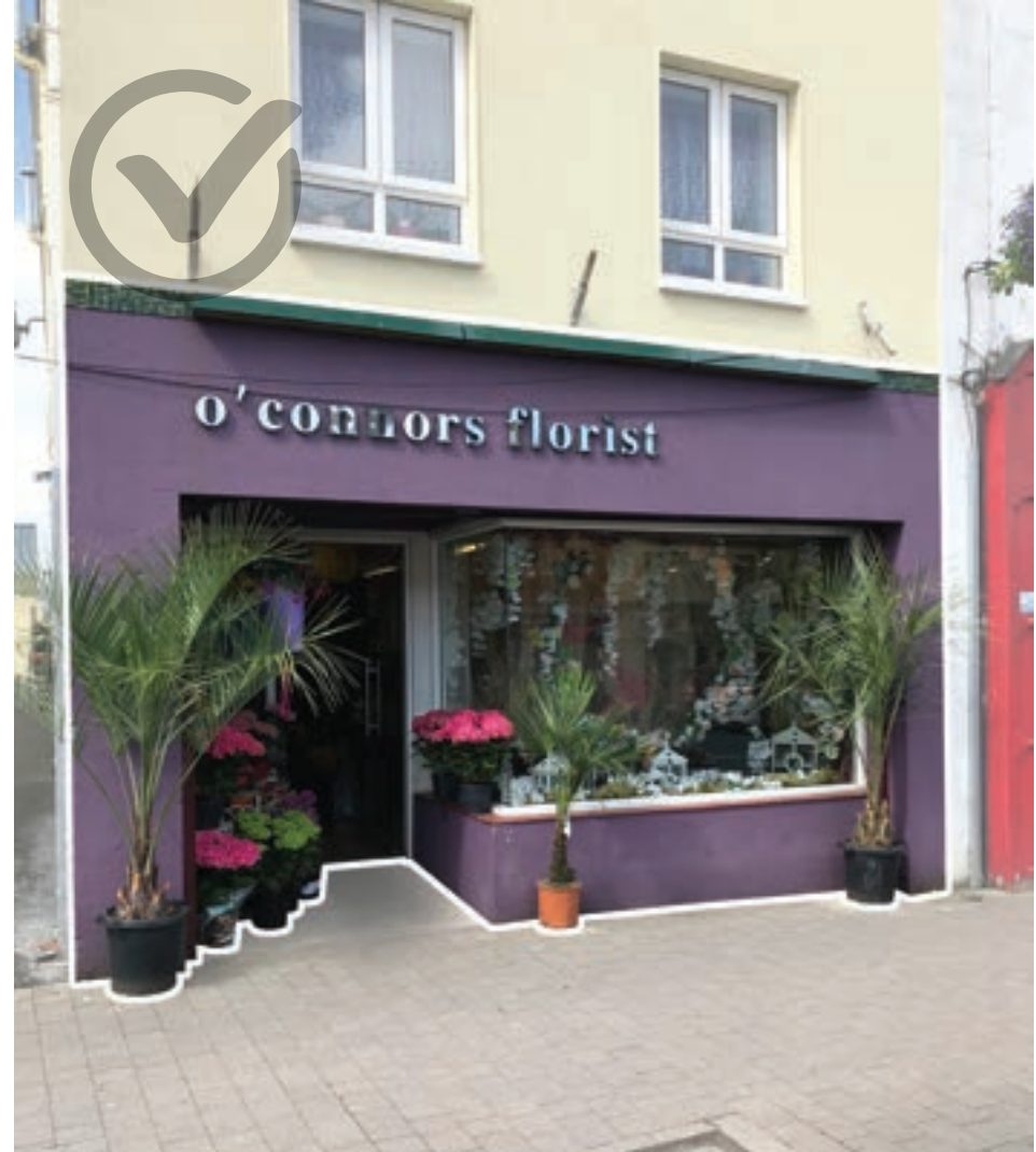
Fig. 38. Neat strip lighting over individual lettering.
