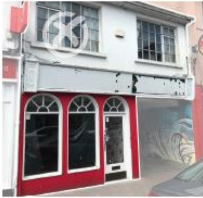
Fig. 3. Vacant retail premises of poor shopfront design, having ground floor window style, size and position not in keeping with upper floor
