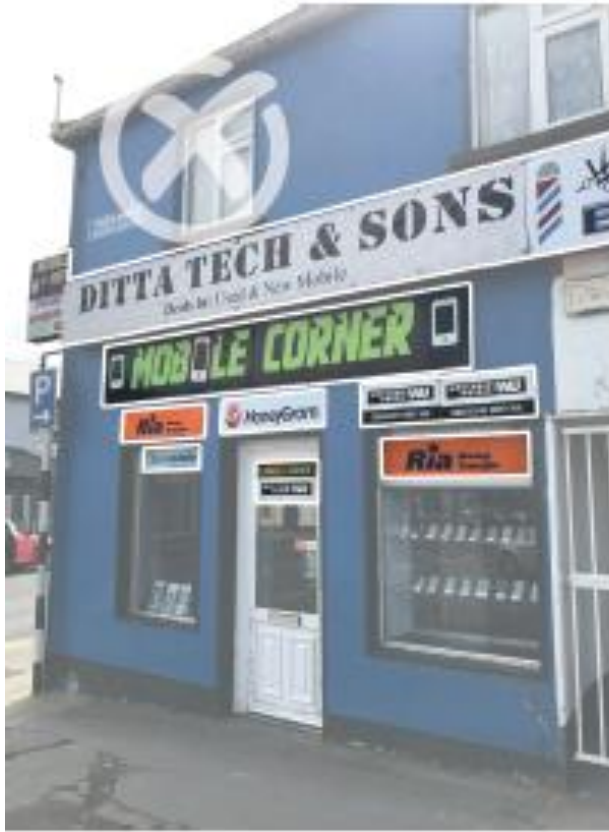
Fig. 12. Excessive signage with double fascia
