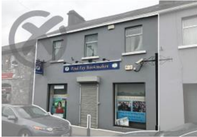
Fig. 22. Bland and uninteresting bookmaker shopfront with unsuitable, externally mounted security shutter and shutter box.
