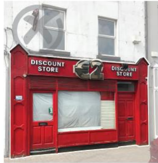
Fig. 30. Disproportionate signage scale and with stunted window and door proportions.
