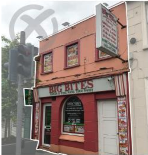
Fig. 29. Excessive number of stickers on shopfront and façade windows.
