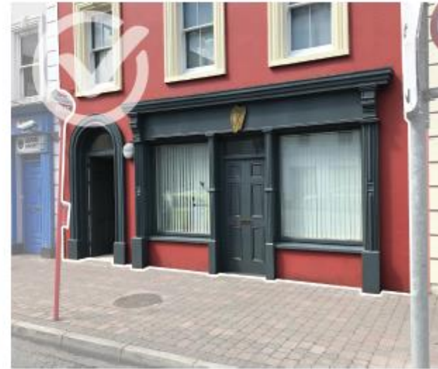
Fig. 31. Simple and consistent shop front colour and signage on a quality timber arrangement.
