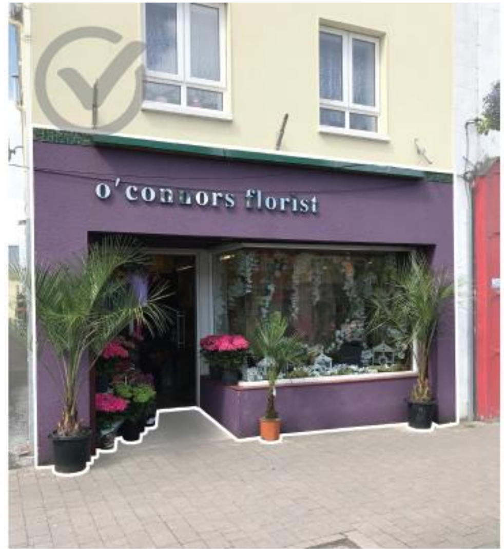
Fig. 38. Neat strip lighting over individual lettering.
