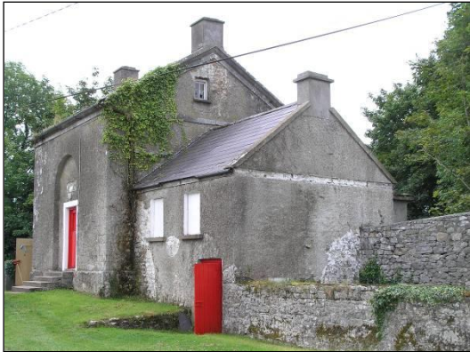
The use of brightly painted doors and windows can be used to brighten up a render finish
