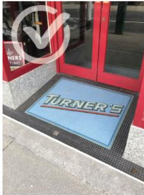
Fig. 6. Recessed doorway with quality threshold finish.
