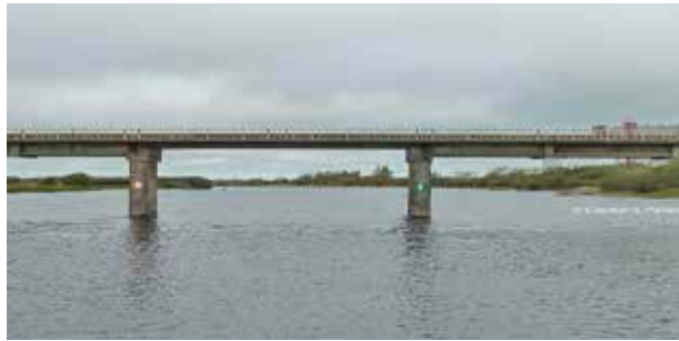
Pic. 10: Bord Na Móna bridge at Lanesboro.
