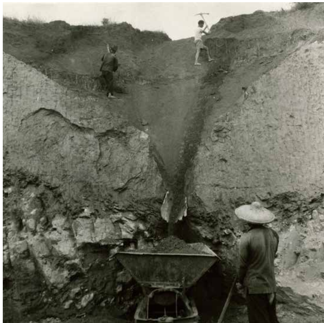
青山陶業的員工從採泥場採挖黏土。攝於 1956。圖片 © 香港大學圖書館。 Mining clay from the quarry to make bricks at the Castle Peak Ceramic Company, 1956. Photo © HKU Libraries.
