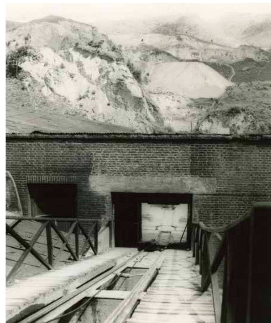
設於青山的鐵道運輸系統，專門用作從採泥場運送黏土到製磚廠。攝於 1956。圖片 © 香港大學圖書館。 System used to transport clay from quarry to brickwork factory in Castle Peak, 1956. Photo © HKU Libraries.
