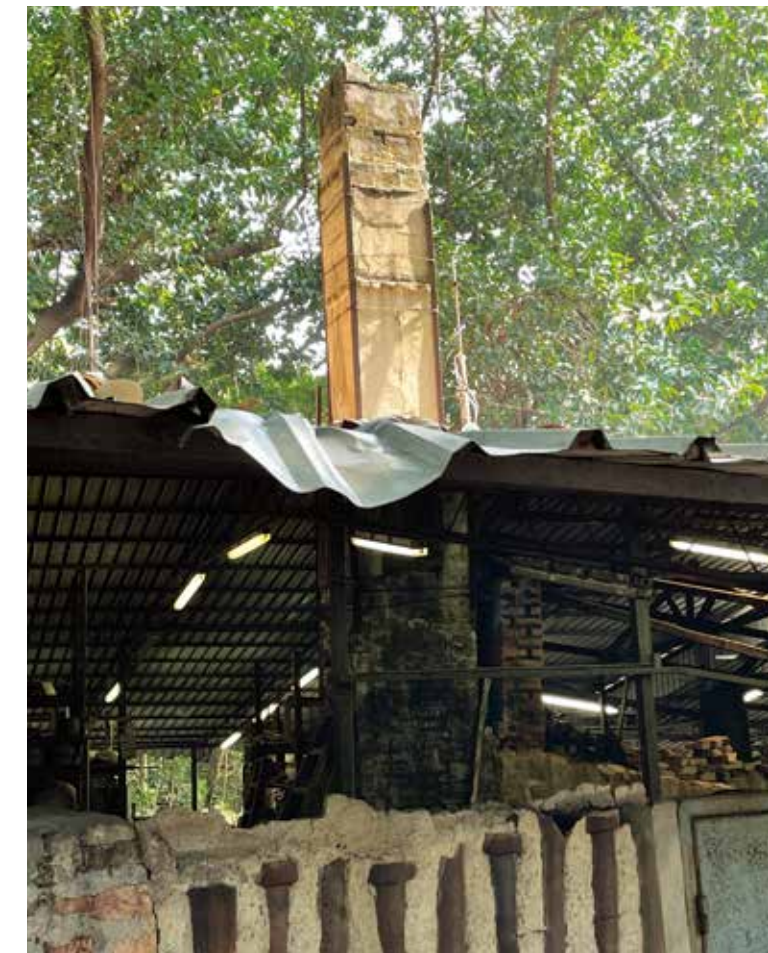
煙囪高 7.65 米，高於窯體其餘部分，能產生強大抽力，把窯頭熱力一直帶到窯尾。 At 7.65 metres tall, the chimney draws the fire along the full length of the kiln.
