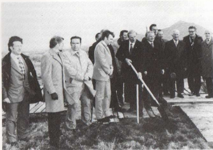
TURNING THE SOD — for the advance factory which is to be built at Cahir. Mr. Denis Gallagher, then Minister for the Gaeltacht, uses the spade.
