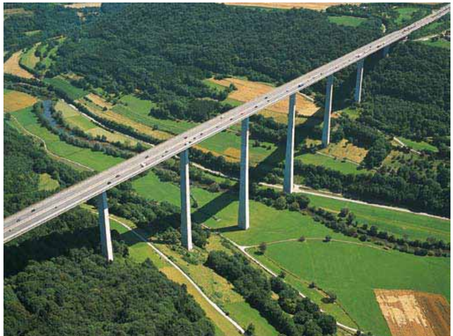
The infrastructure of the state is an important factor for the competitive strength of Baden-Württemberg. The photo shows the Kochertal bridge at Braunsbach-Geislingen near Schwäbisch Hall, Germany's highest motorway bridge.
