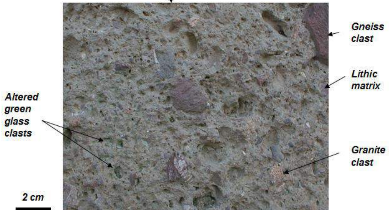
Figure 27: Chassenon Roman church built in suevite (suevite sensu stricto) and close up view of the wall
