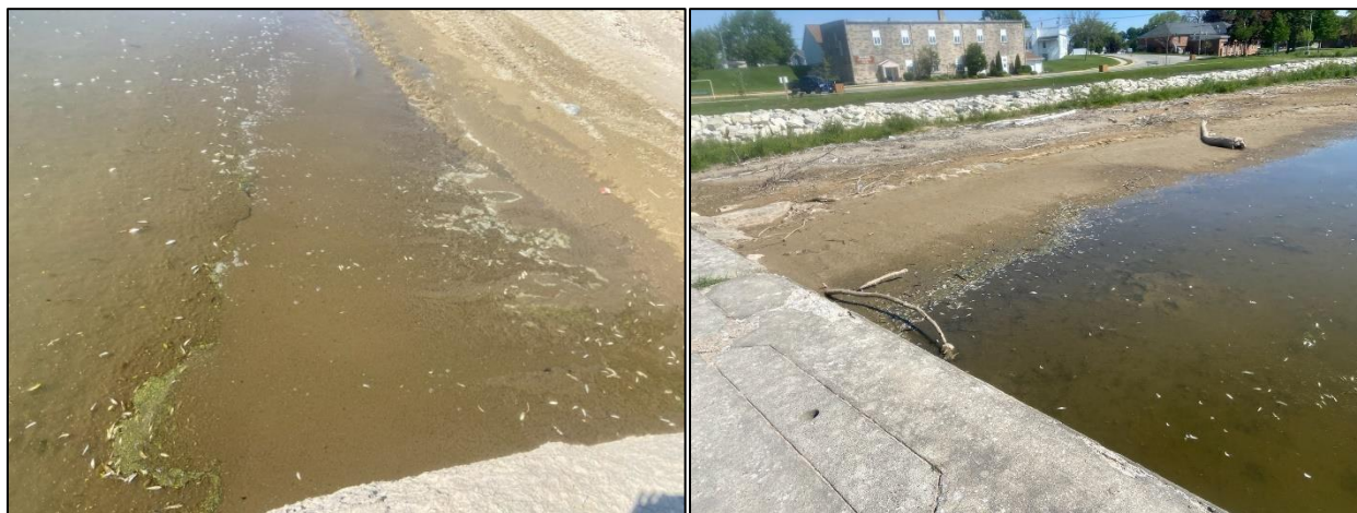
Photo 3: Evidence of collection of detritus as the point where the south breakwater meets the shore. Left - Lakeward side. Right - Harbor side. Photos taken July 2022.
