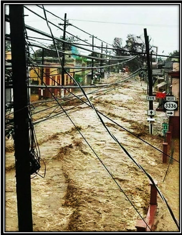
Photo 2: Road PR-127 Becomes Flood Diversion Channel for most Floods
