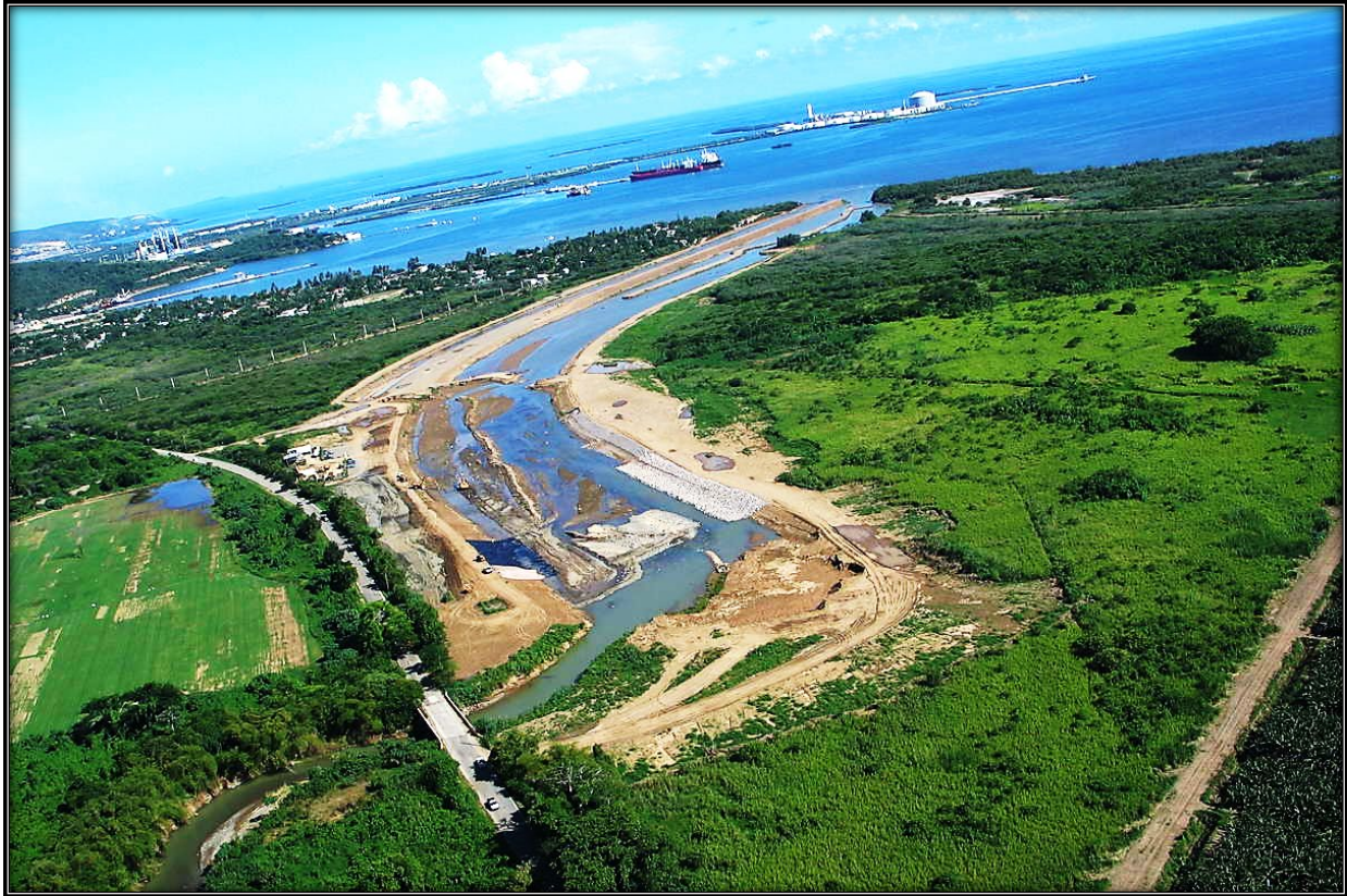
Photo 1: Phase I Construction Activities
