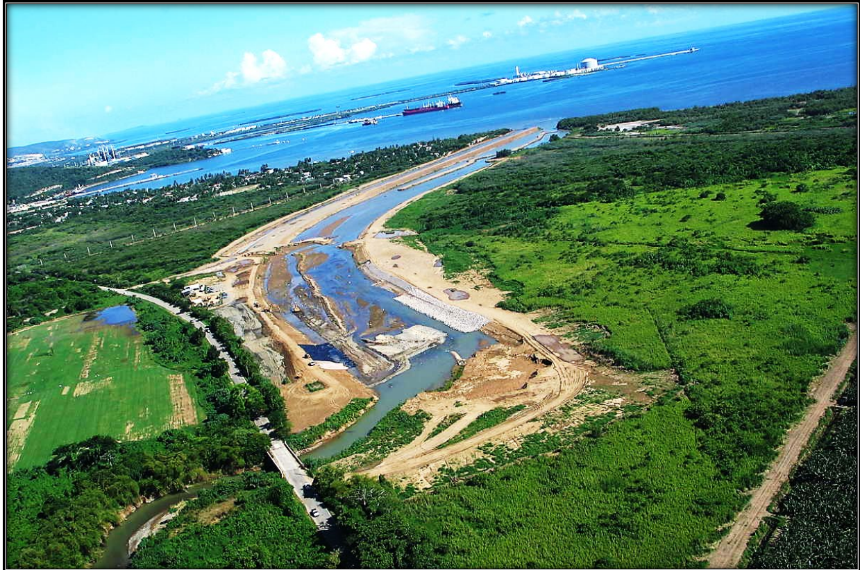
Photo 1: Phase I Construction Activities
