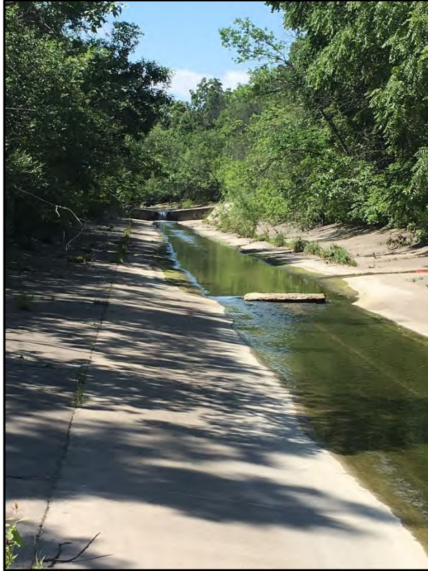
Figure 9 – View of typical Honey Creek streambed throughout the project reach.
