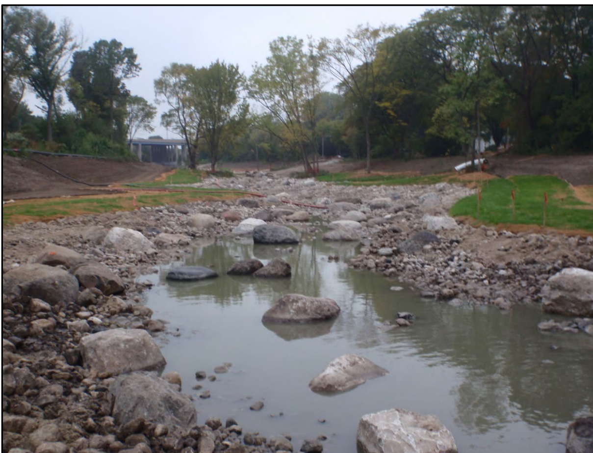
Figure 14 – Example of Reestablishment of Floodplain Connectivity, Underwood Creek, WI Section 506
