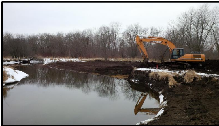
Figure 32 Grading Riverbank to Mimic Natural Shapes and Morphology
