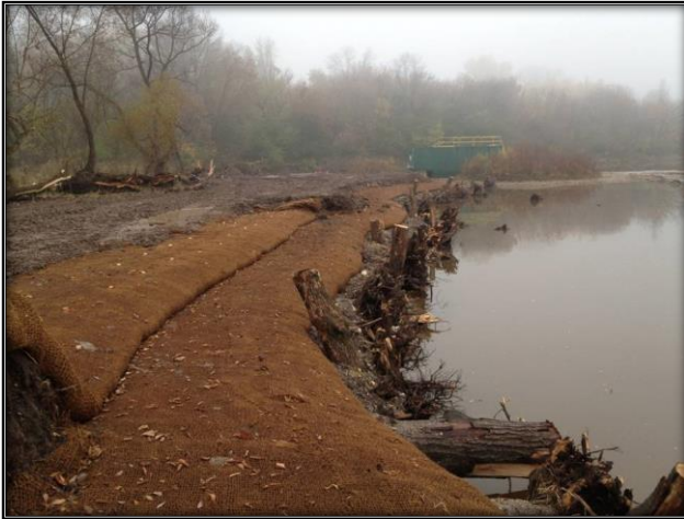
Figure 34 Large Woody Debris Structure and Soil Terracing
