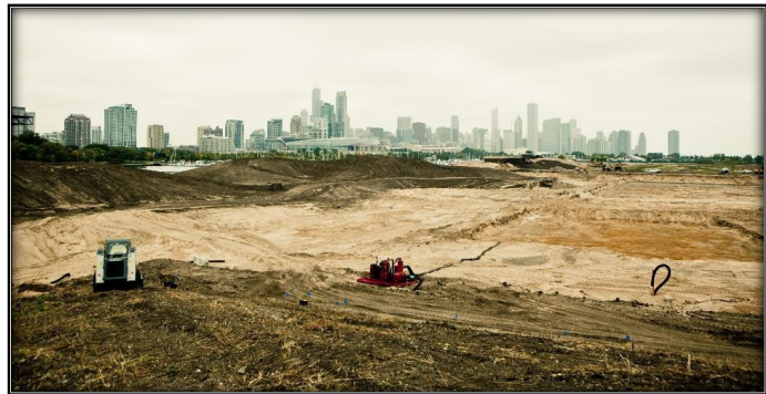
Figure 31 Excavation of Lagoon
