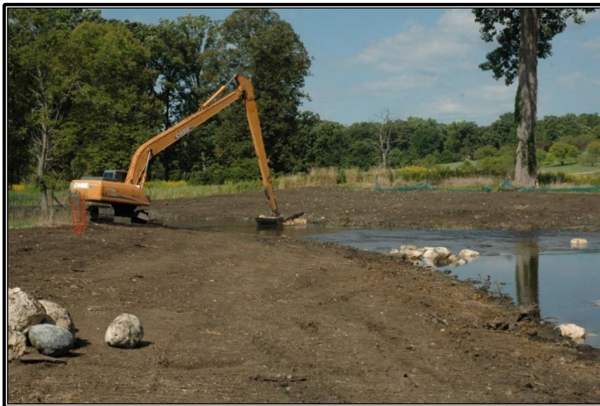
Figure 44 Example of excavation of a basin/swale structure
