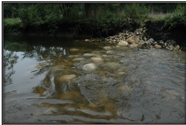
Figure 33 Boulder and Cobble Riffle Placement
