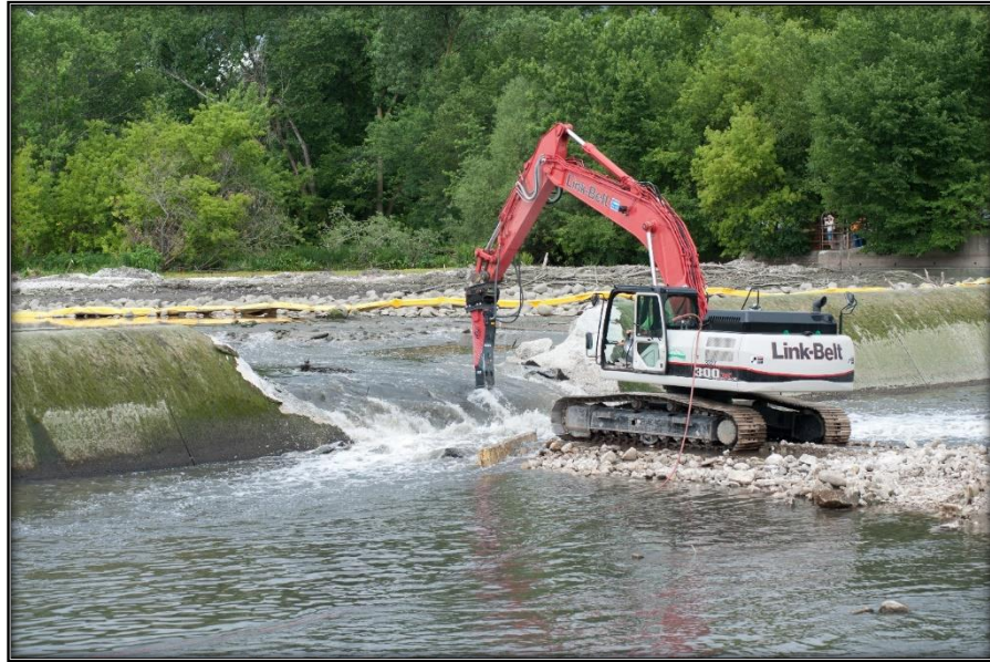
Figure 30 Demolition of a Low Head Dam
