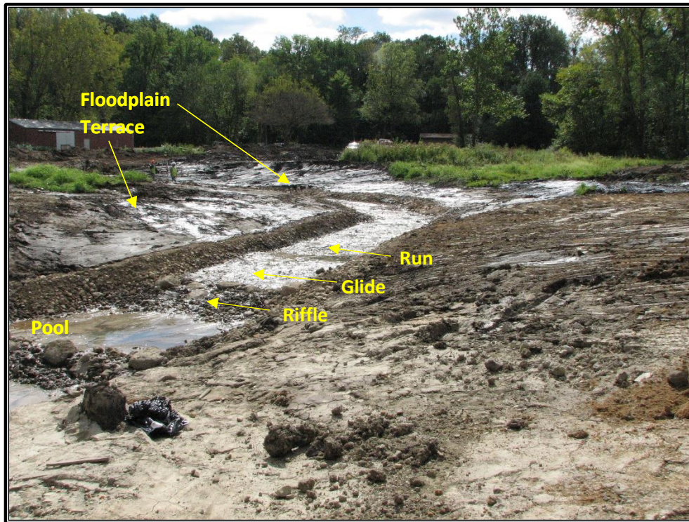
Figure 43 Example of Stream Sculpting on Little Calumet River at Red Mill Pond ER
