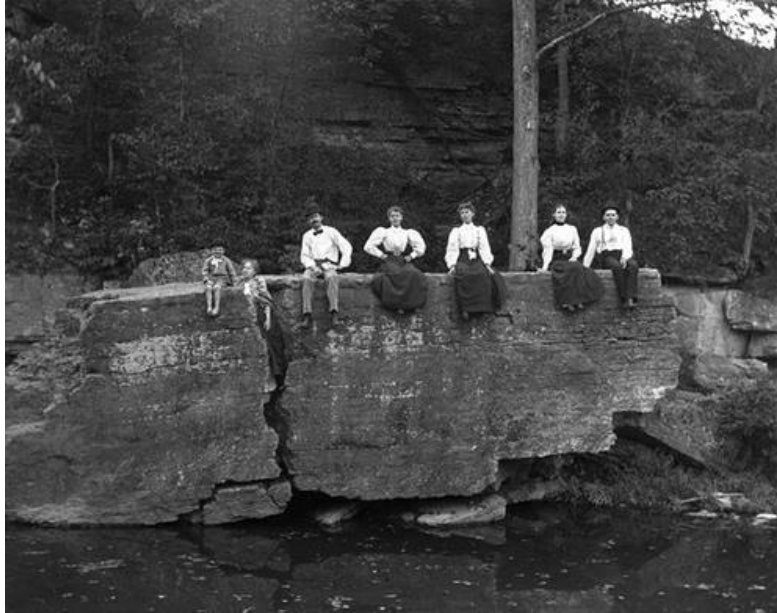
Figure 1 Big Rock at Cherokee Park in 1936. Photo credit - The Olmsted Conservancy
