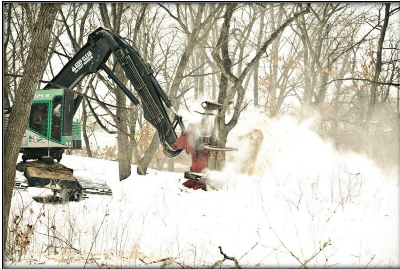
Figure 36 Removal of Cottonwoods and Ash from Globally Imperiled Ridge and Swale
