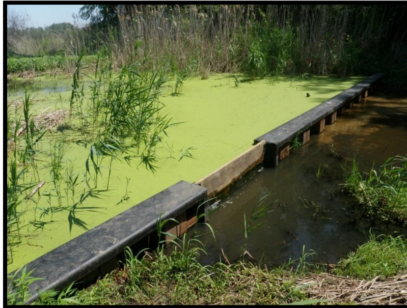
Figure 35 A Water Control Structure Used to Stabilize Hydroperiod as part of the Chicago District's Indian Ridge Marsh Ecosystem Restoration in Chicago, IL.
