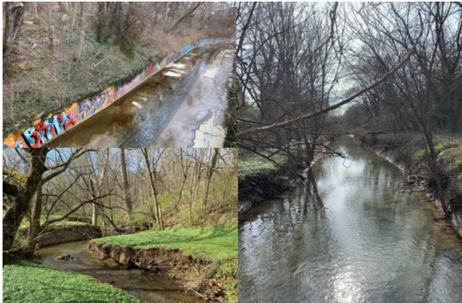
Figure 21 Example of common problems seen in Beargrass Creek. Top left- concrete channel on the South Fork, Bottom left- Channel incision on the Middle Fork, and Right- Channelization and loss of riparian zone on the Muddy Fork
