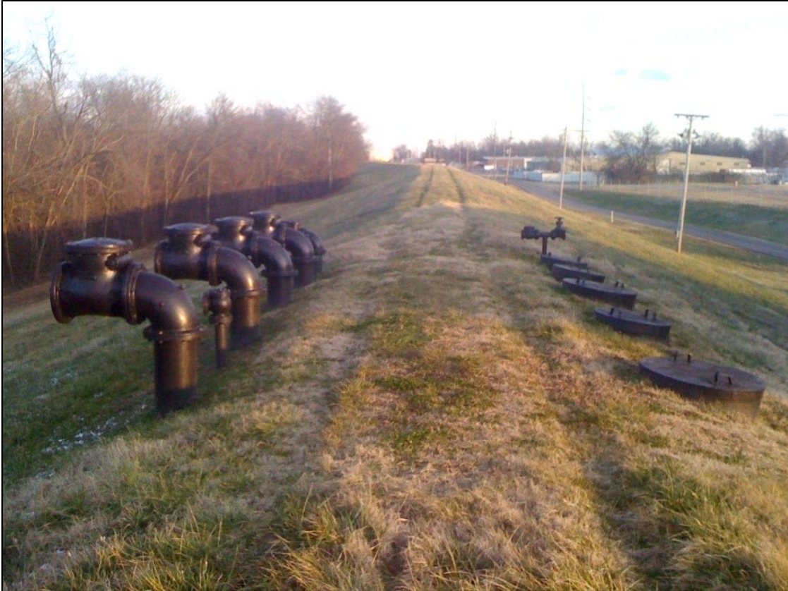
Figure 6-11. Potential inspection access points for pump station discharge pipes.
