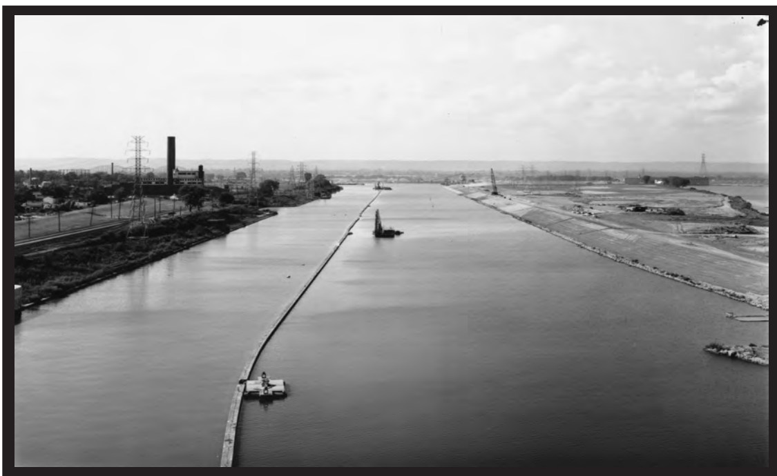
Downstream view from Ohio Falls (Pennsylvania Railroad) bridge of the canal widening in 1960. The old canal wall has not yet been removed, indicating the old 200-foot canal width. (Corps of Engineers)
