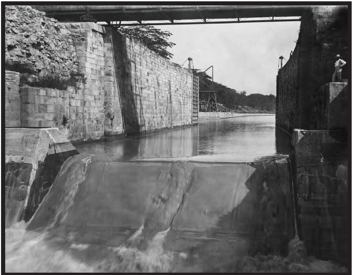
Captain Hiram Chittenden designed a beartrap gate installed in the original locks of 1830. It began operation in 1899 to flush mud from the locks and canal into the river below. (Corps of Engineers)
