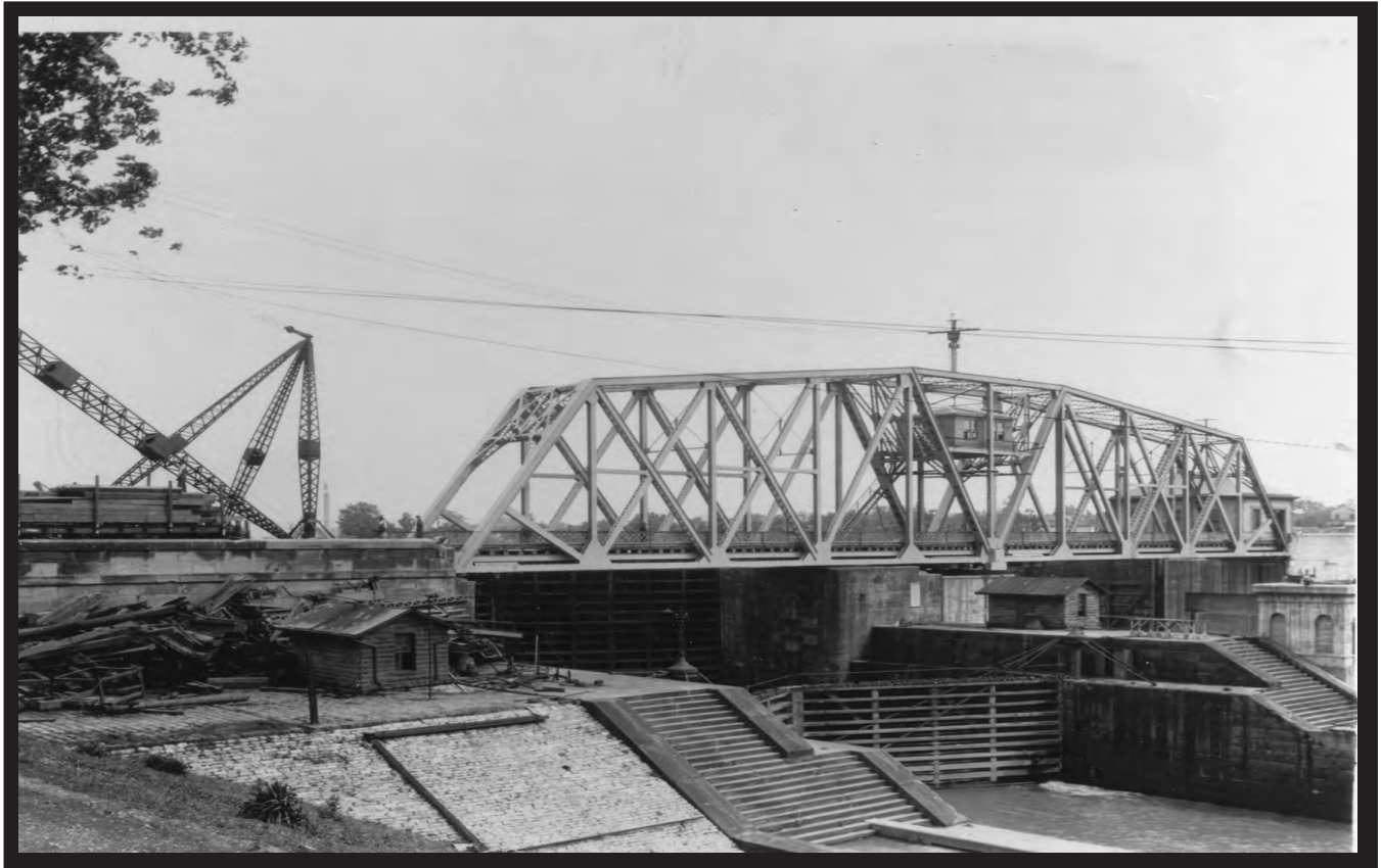
A May 1926 view of the combined railroad and highway bridge placed over the locks by the power company. Scowden locks are in the foreground and Lock 41 is in the back at the right. (Corps of Engineers)
