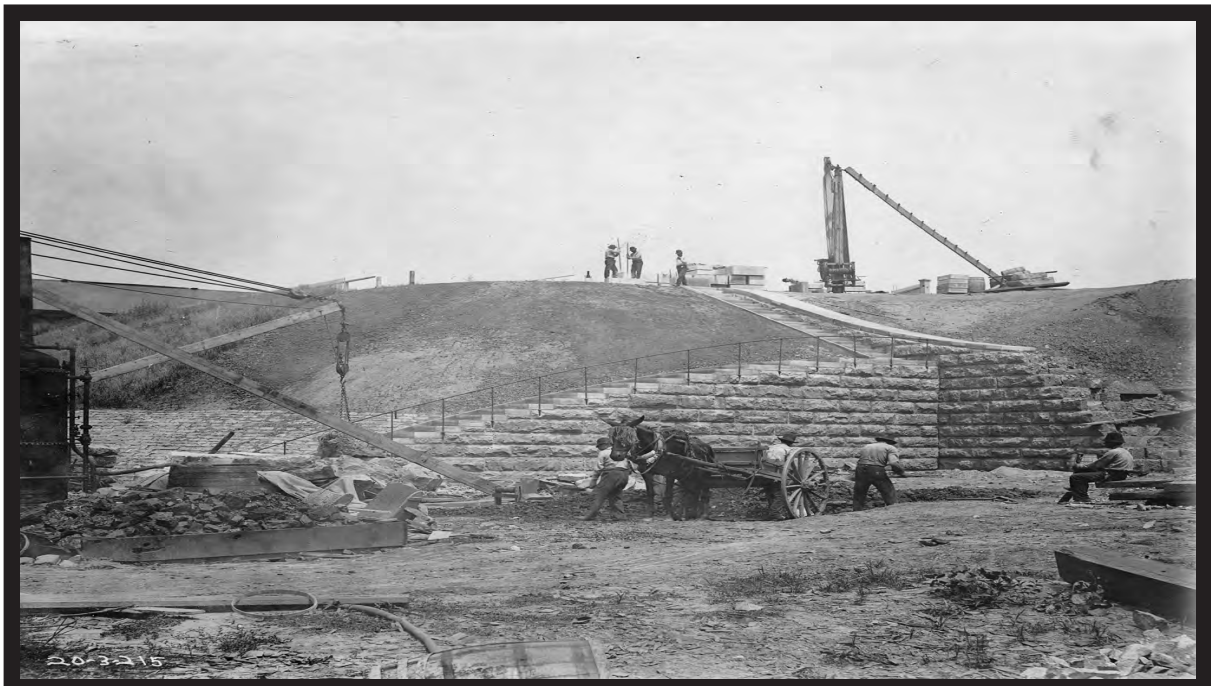
Both steam and mule power was used to finish the canal. (National Archives)
