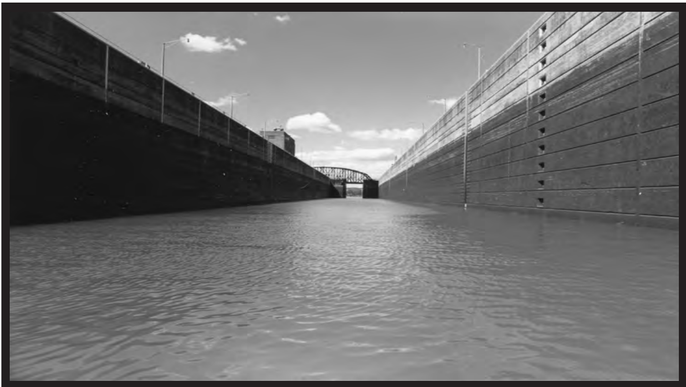
A 1988 view inside the 1200-foot McAlpine Lock with lower lockgates opening. (Corps of Engineers)
