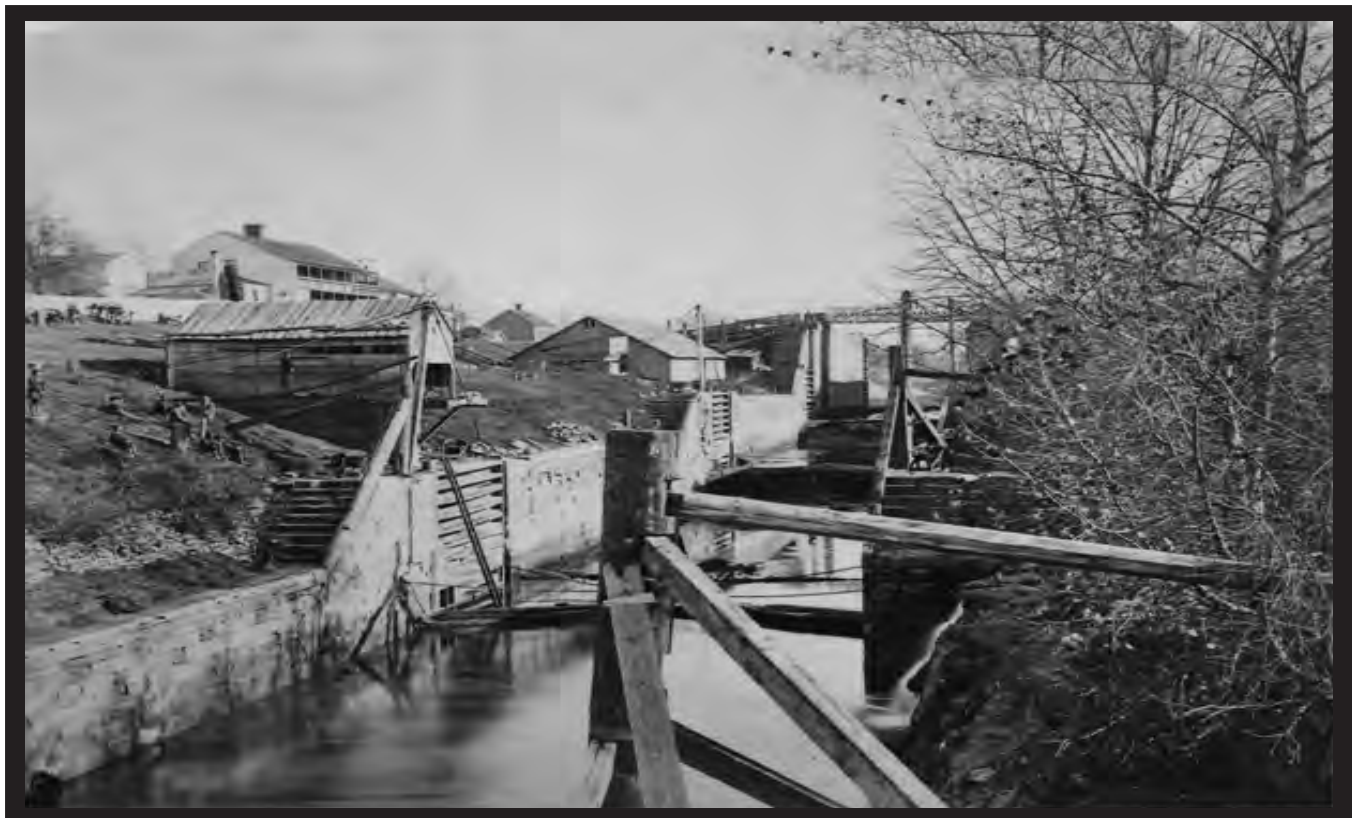
Lockmen walked in circles to turn capstans, winding up chains to open or close the lock gates. (Corps of Engineers)
