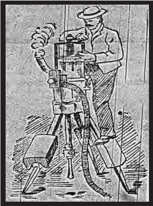
Steam drills supplanted manual drilling for rock excavation during the 1860s. The drilled holes were loaded with explosives and detonated to shatter the rock. (Courier-Journal)
