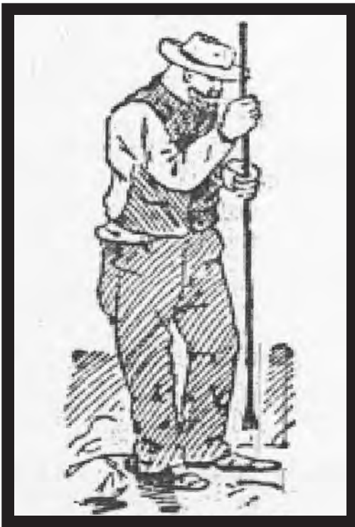
To excavate rock from the canal, men drilled holes by hand that were filled with gunpowder and detonated. (Courier-Journal)
