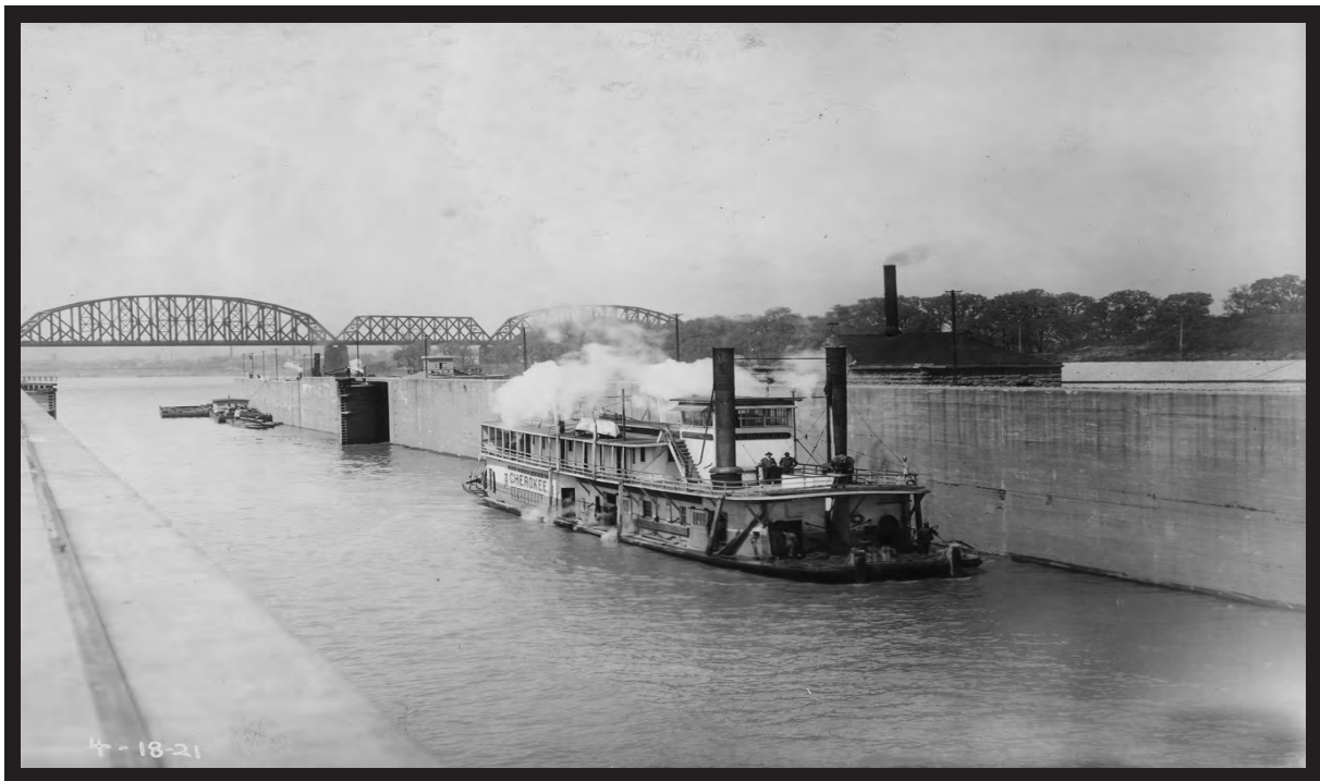
The Corps towboat Cherokee made the first test lockage at Lock 41 on April 18, 1921, and the new 600-foot lock officially opened to commercial traffic on May 1. (Corps of Engineers)
