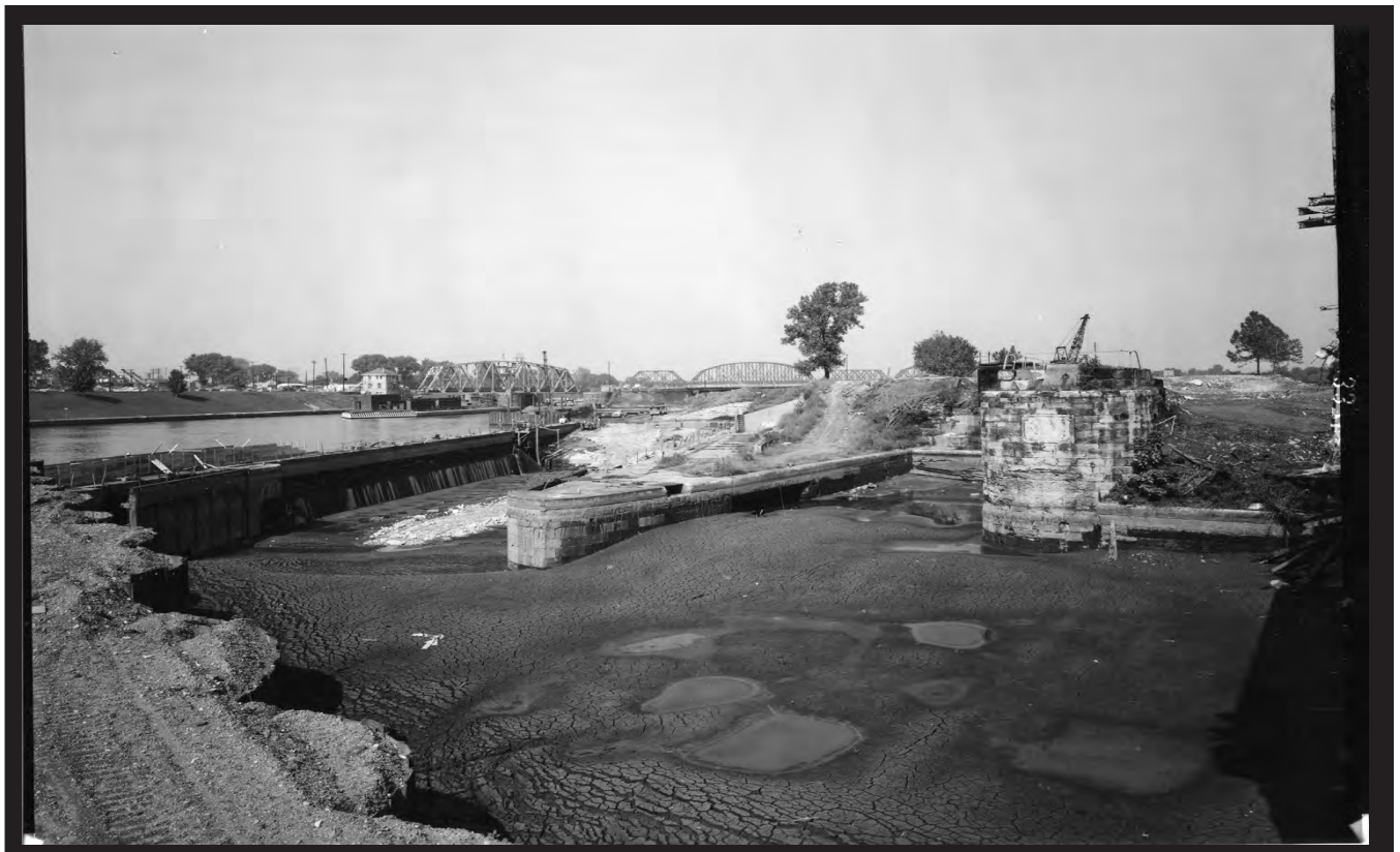
This 1959 view shows mud filling the old dry dock. (Corps of Engineers)
