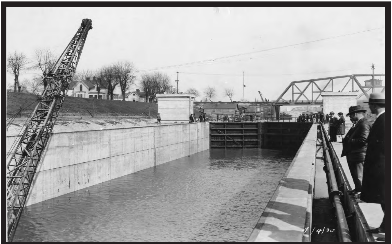
Onlookers on April 4, 1930, watch for a boat to make the first lockage through the new auxiliary lock built in the lower chamber of Scowden Locks. (Corps of Engineers)
