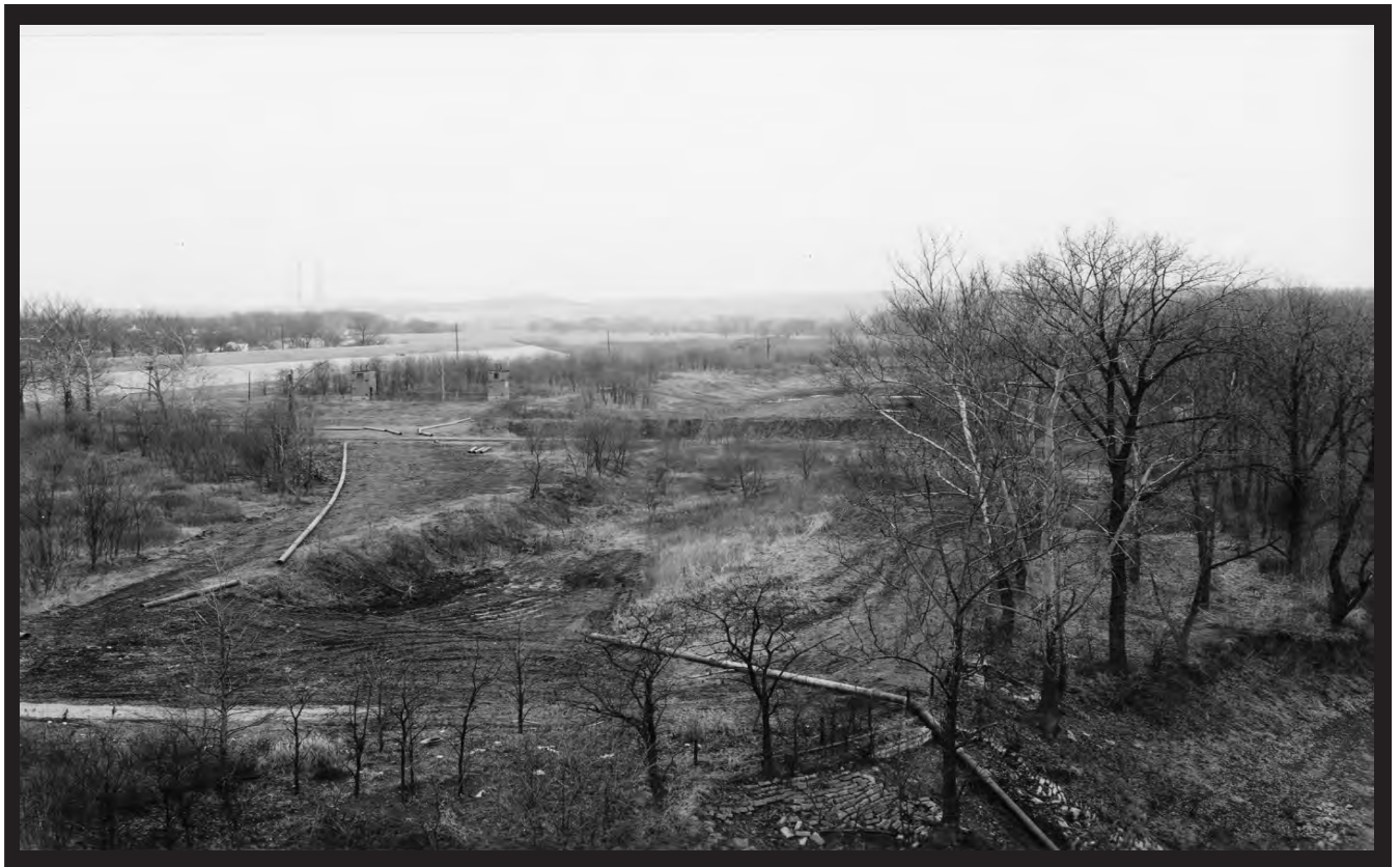
Materials excavated from the canal basin were pumped through these pipes to create fill along Portland wharf. (Corps of Engineers)
