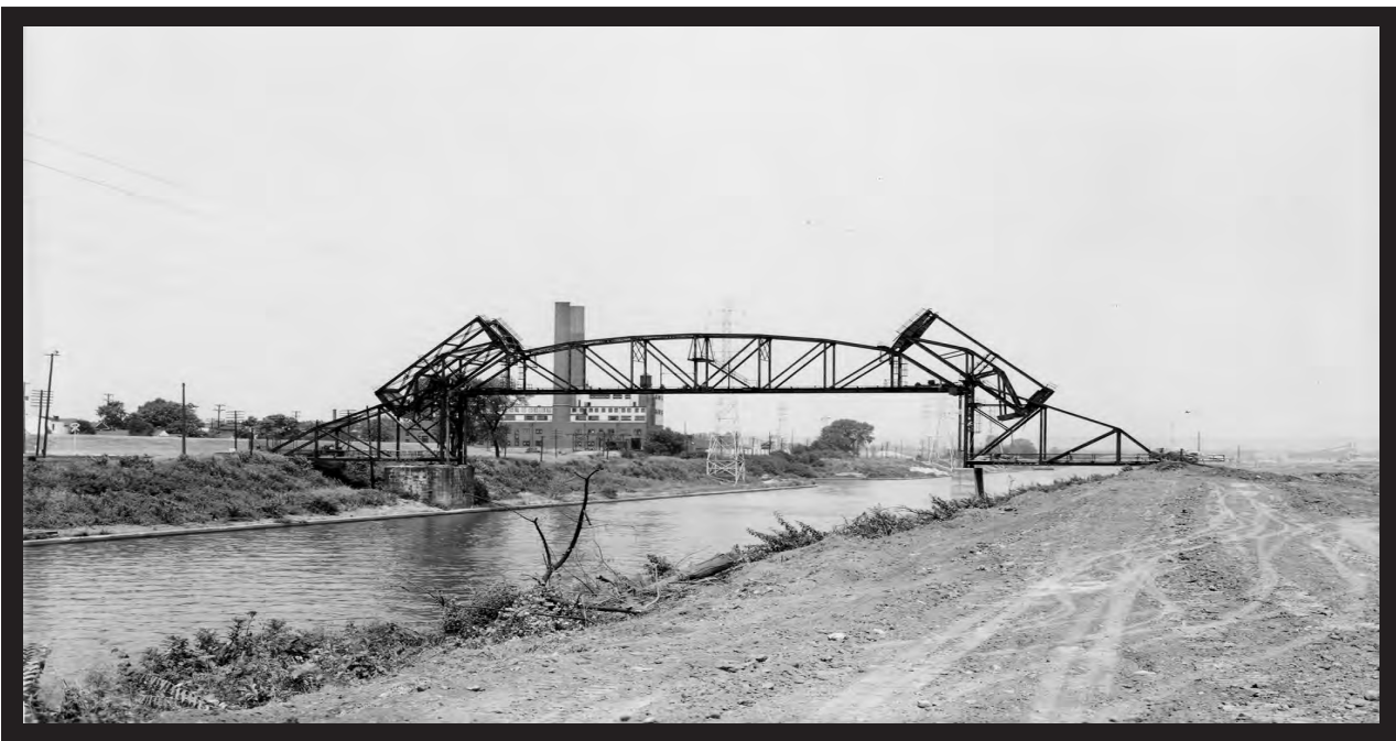
Downstream view of the Eighteenth street bridge just before its removal in 1959. Excavating on the right or north side widened the canal from 200 to a 500-foot width, also removing the former site of the Elm Tree Garden. The pier on the left or south side remained and in 1999 became the base of an overlook on the municipal Riverwalk. (Corps of Engineers)
