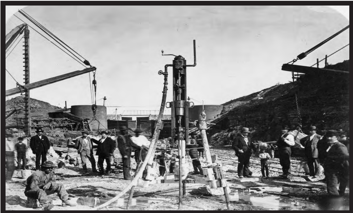
Reporters observe the excavation of Scowden locks. (Corps of Engineers)
