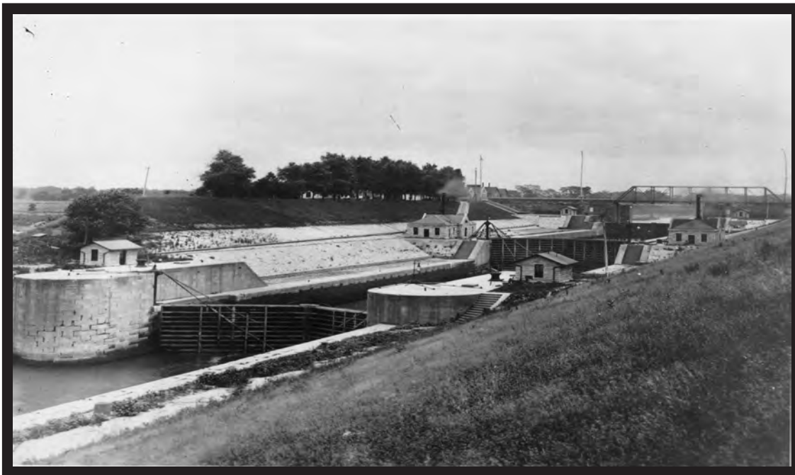
Scowden locks during construction and as they appeared at their completion in 1872. (National Archives)
