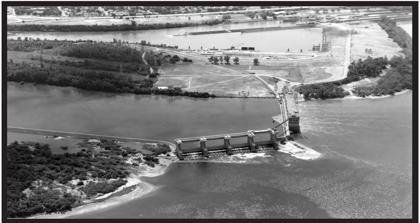
Aerial view of the four lower Tainter gates next to the hydroelectric station. They are closed against the sills and holding the pool at elevation 420. In the background is the L-shaped remnant of Shippingport island and a barge tow approaching the McAlpine Lock. The filled site of Shippingport village was on the right along the road from the locks to the power station. (Corps of Engineers)
