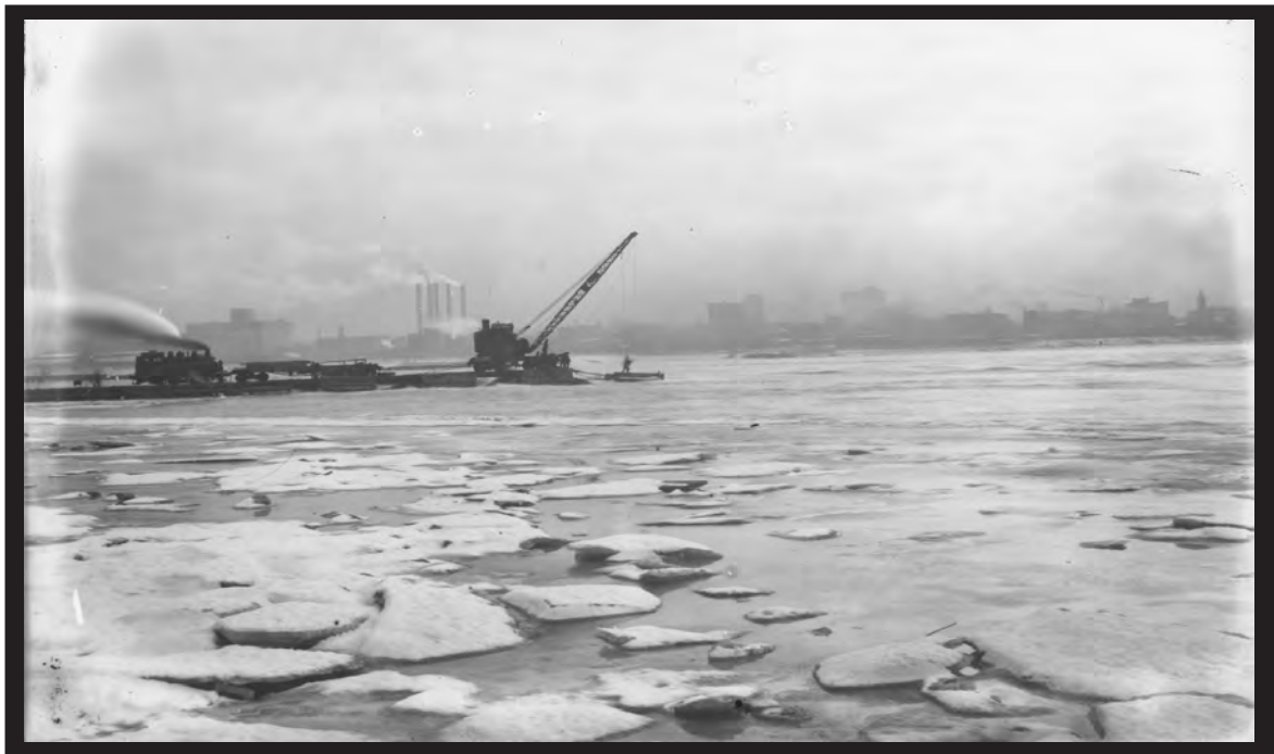
Coal smoke haze hangs over Louisville in early 1926 while a box crane lowers a wooden box into place as the locomotive on the left brings stone to fill the box. (Corps of Engineers)
