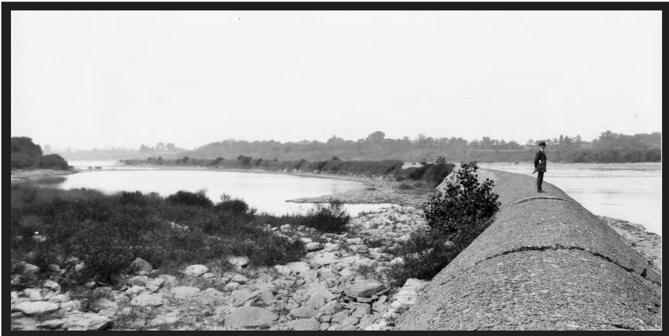
Concrete dikes were built along both sides of Indian chute to confine river flow and boats to the channel. Goose island is behind, to the left, of this dike, and Indian chute is on the right side. (University of Louisville Photographic Archives)
