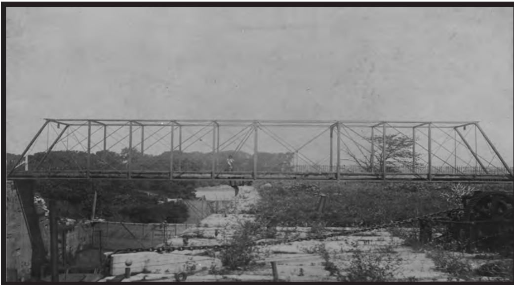
The swing bridge crossed traffic over the locks between Portland and Shippingport. (Corps of Engineers)
