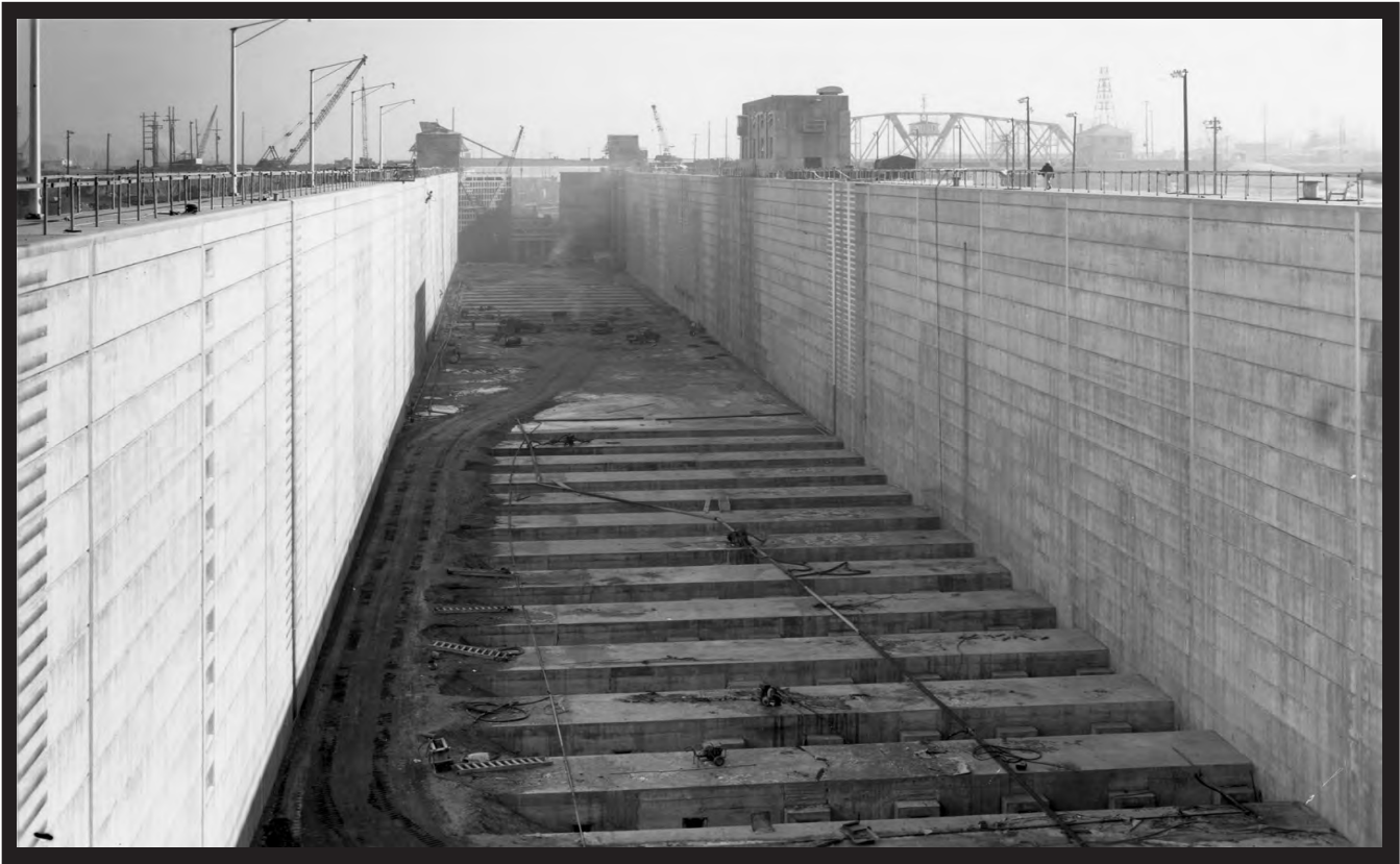
The nearly completed 1200-foot McAlpine Lock in January 1961. (Corps of Engineers)
