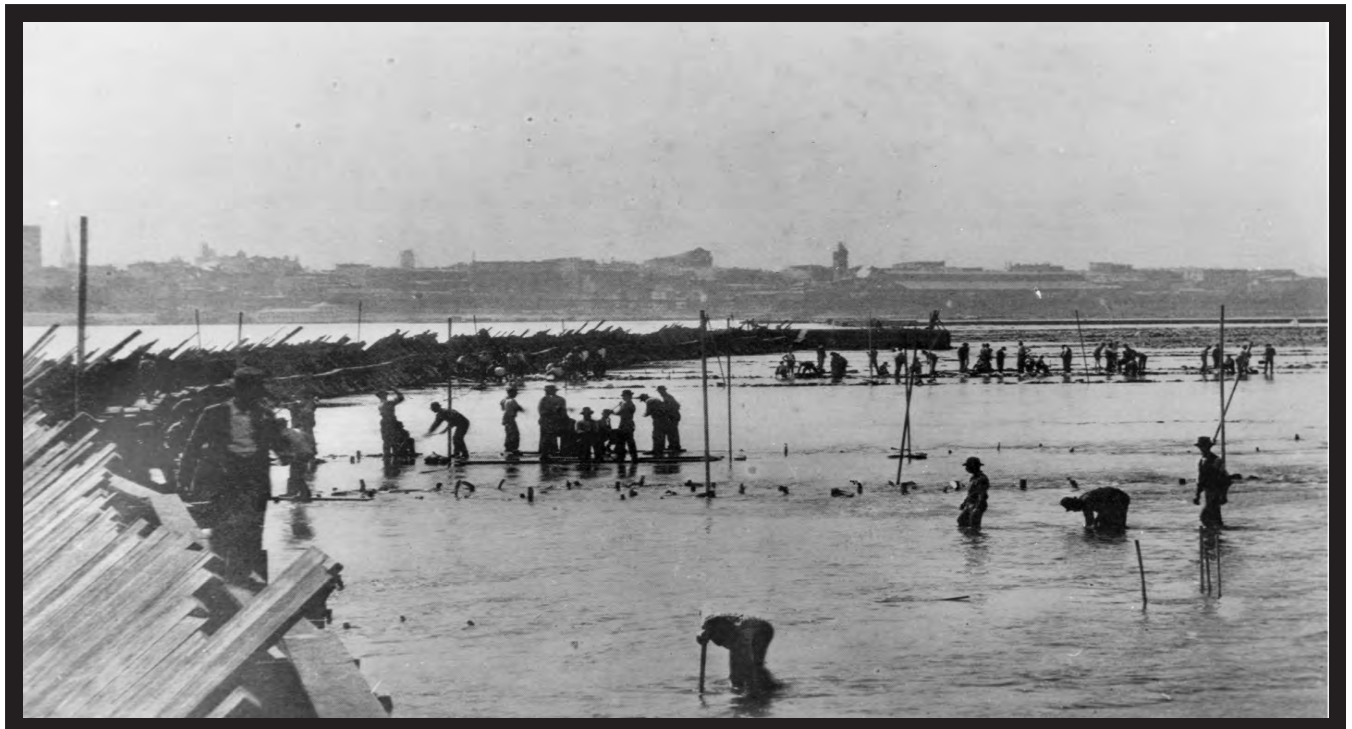
Temporary dams across the head of Indian chute allowed drilling and blasting to proceed. (Corps of Engineers)
