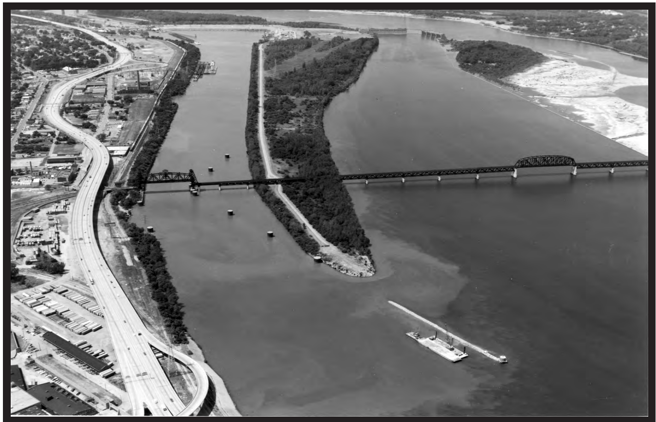
Construction of the vane dike (straight white line of rock) above the head of Shippingport island in 1976 to help prevent the current from sweeping barges down Kentucky chute to the hydroelectric station. At 241-foot width, the space under the railroad lift bridge in the canal is the narrowest passage on the Ohio River, requiring only one-way barge traffic. (Corps of Engineers)
