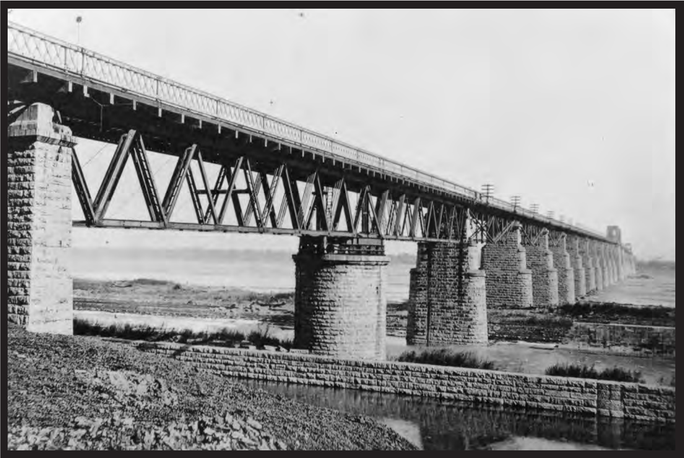
The Ohio Falls bridge at Fourteenth street, designed by Albert Fink and completed in 1870, was the first bridge between Louisville and Jeffersonville. In the foreground is its turnspan over the canal supported by the round pier. (University of Louisville Photographic Archives)
