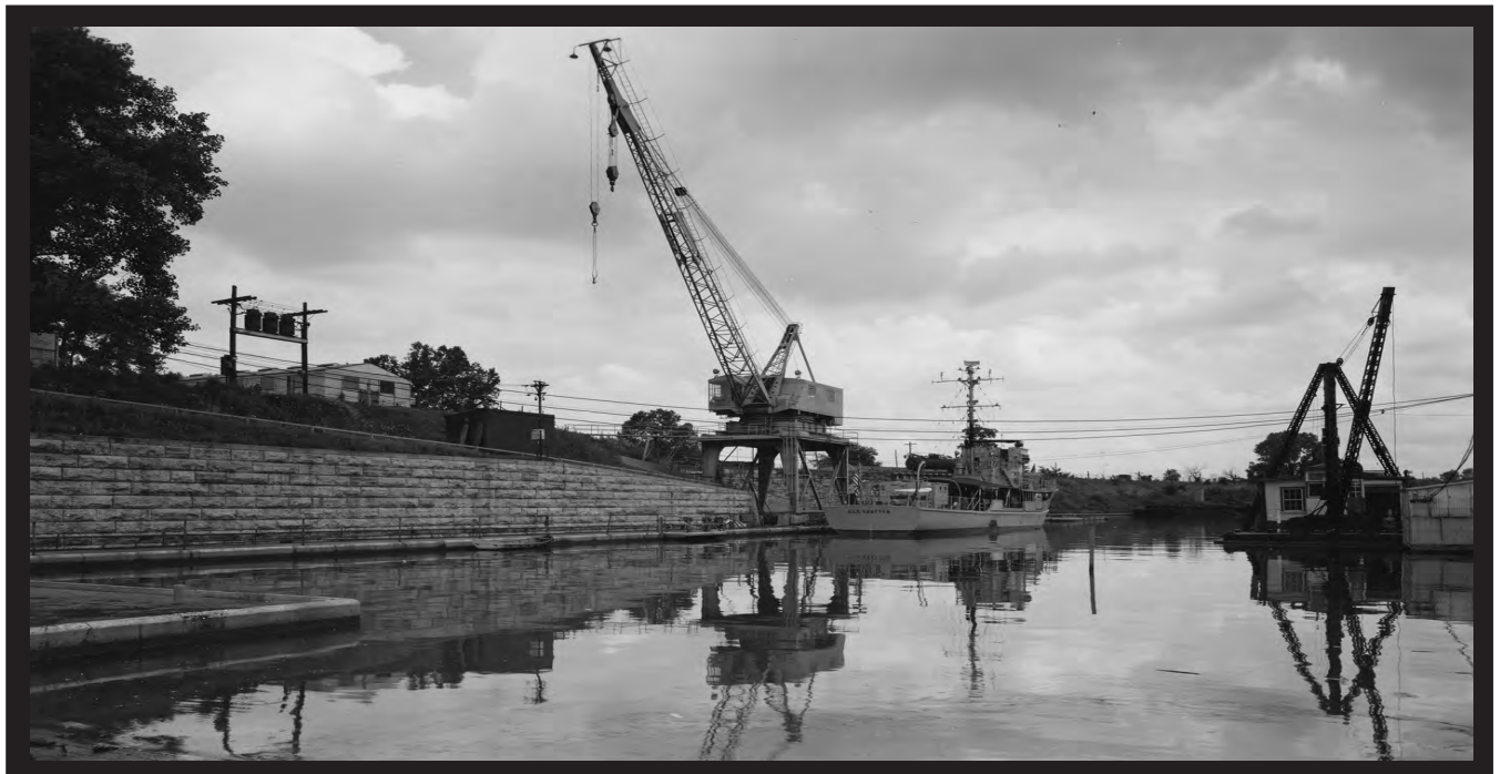
Many warships built on the Ohio passed through the canal on the way to overseas service during the Second World War, but few photographs of them exist because cameras were banned for security reasons. This ship, the U.S.S. Grafton , moored in the canal during postwar years for training use by the Navy Reserves. (Corps of Engineers)
