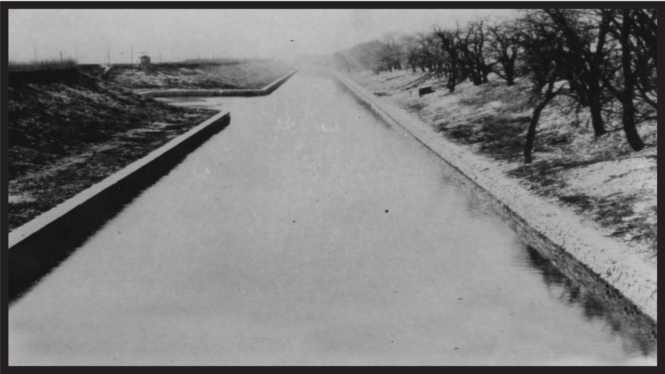
The widened canal had turnout basins to allow boats to pass while in the canal. (Corps of Engineers)
