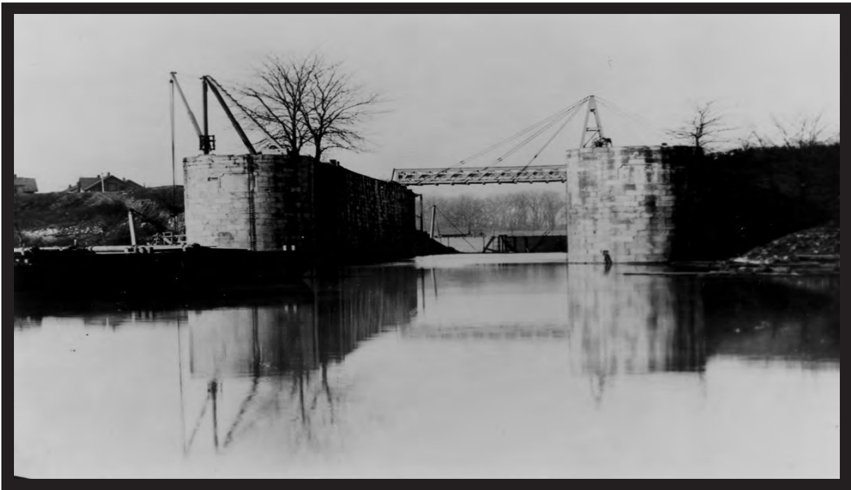
The guard gates at the head of the canal had a bridge that could be swung aside for boat passage. (Corps of Engineers)
