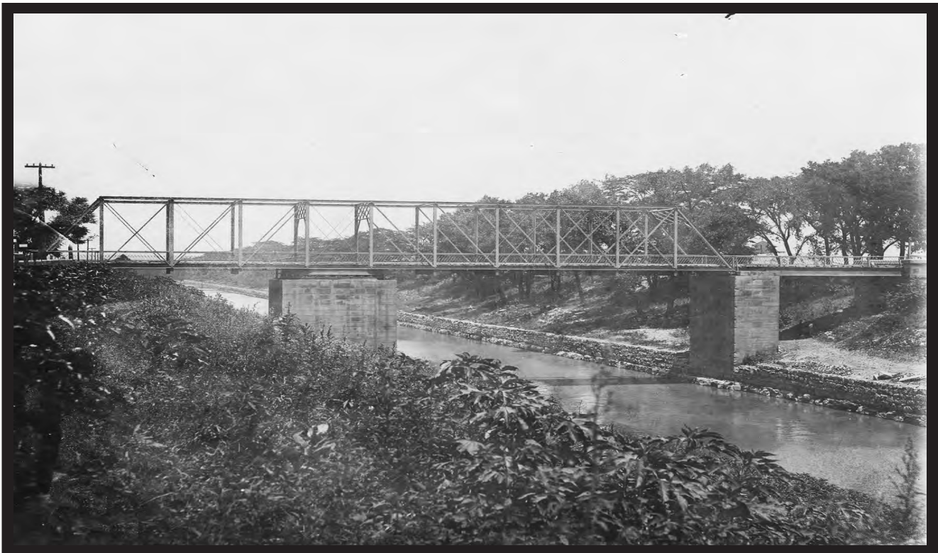
Although Frank McHarry and Shippingport residents opposed it, this pivot bridge replaced the stone arch bridge across the canal at Eighteenth street in 1856. (Corps of Engineers)
