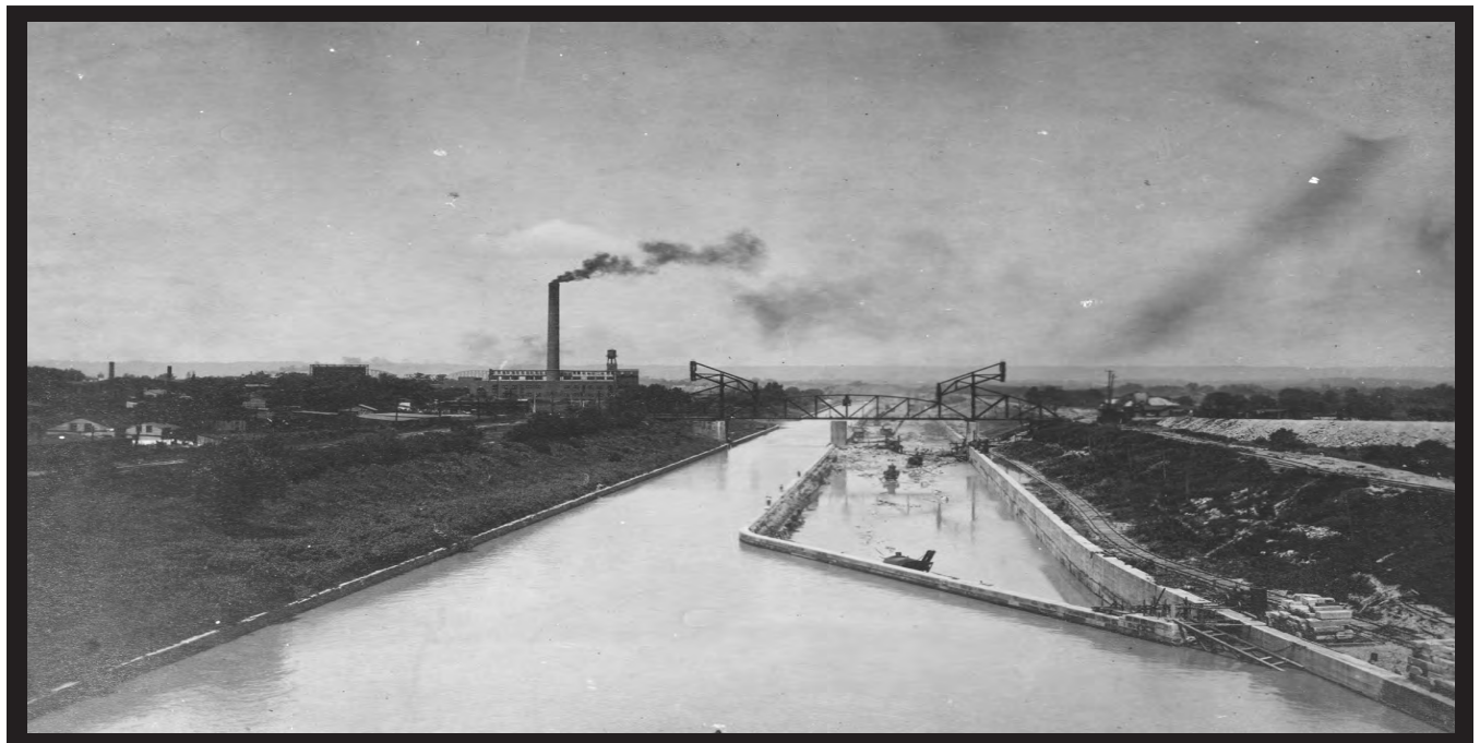
The old canal wall was left in place while the canal was widened to 200 feet behind the wall. (Corps of Engineers)
