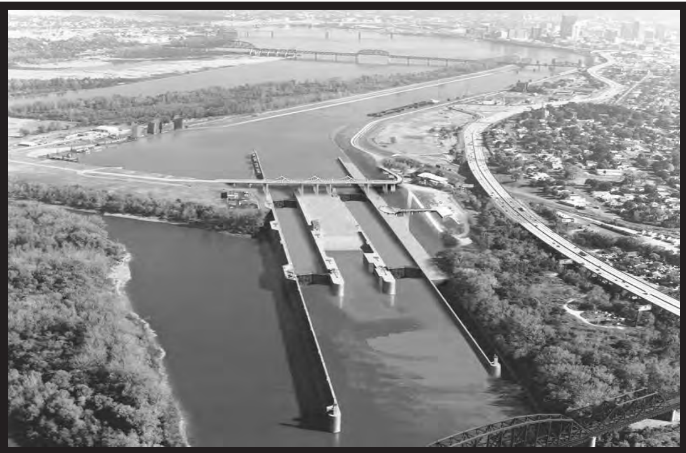
Rendering of the completed McAlpine Lock Project.
