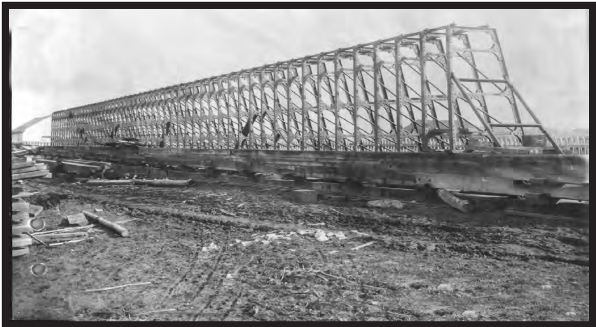
General Weitzel adopted the Boule movable dam, invented in France, to control river flow over the Falls. The metal trestles were manufactured and assembled at the canal repair station, then installed in the dam at the crest of the Falls. (National Archives)
