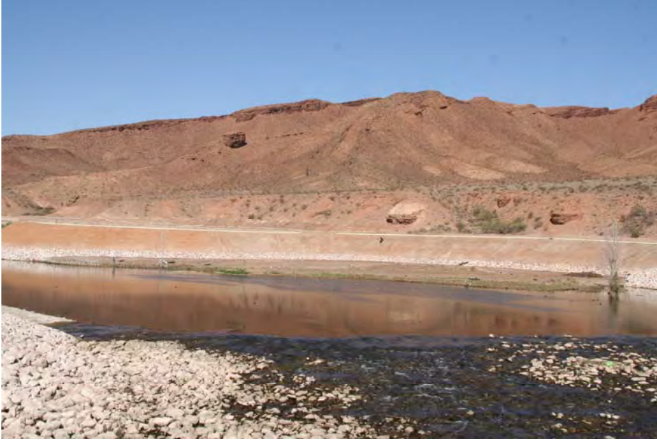
View of the Powerline Crossing Weir with riparian and upland planting sites viewable in the background.
