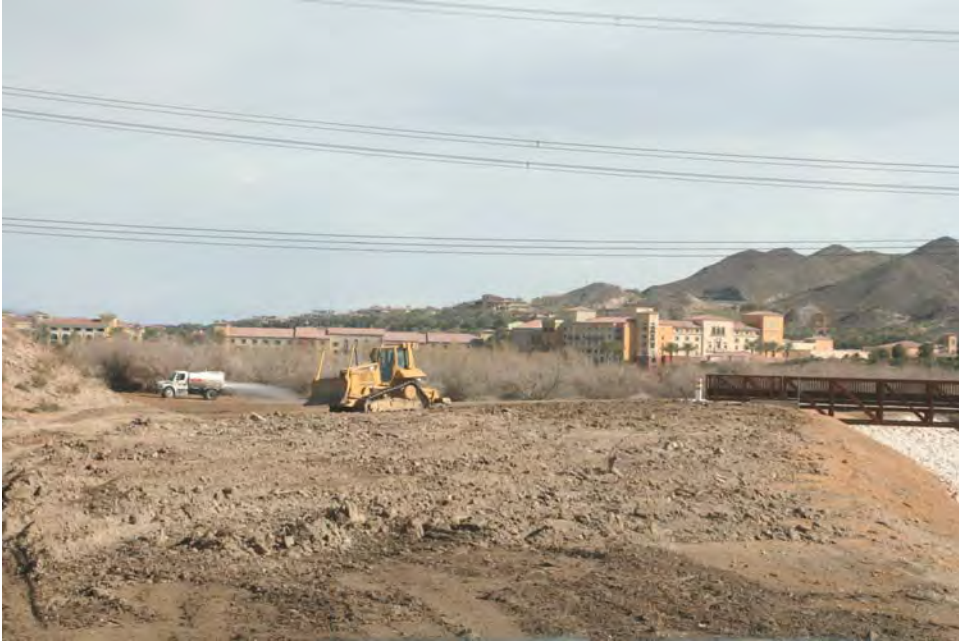
Dozer and water truck tilling an upland site prior to revegetation.
