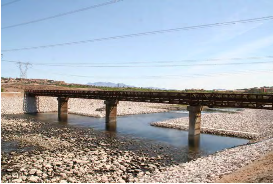
Hardstem bulrush material planted on the Powerline Crossing Weir.
