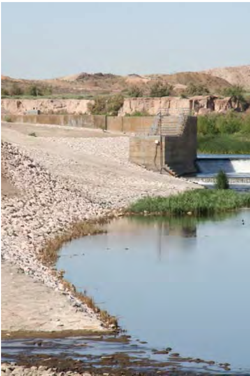
Hardstem bulrush (brown material in the foreground) planted along bank protection.
