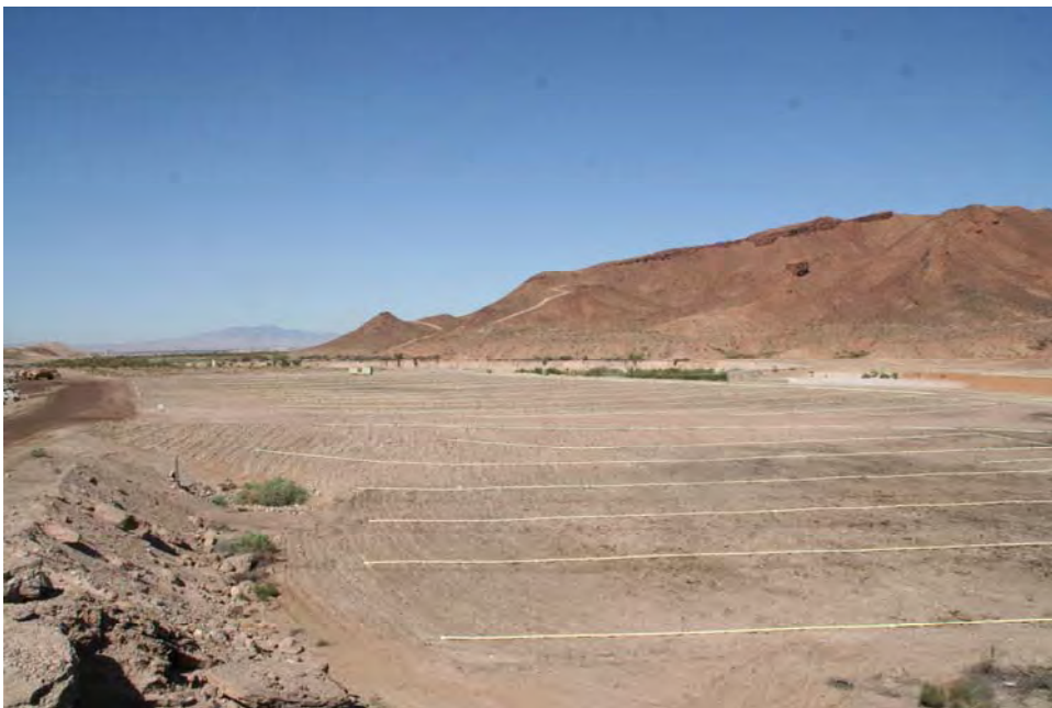
Irrigation system installed on an upland planting matrix.
