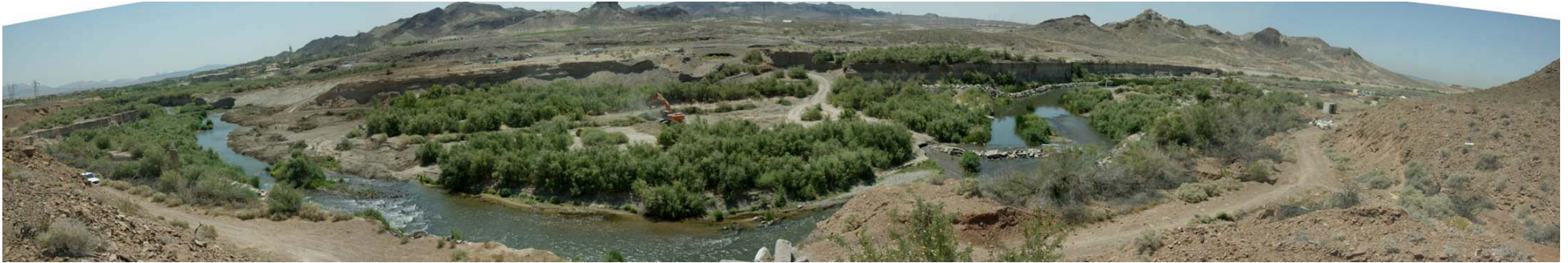
June 2003 image of the Rainbow Gardens weir location (prior to construction)
