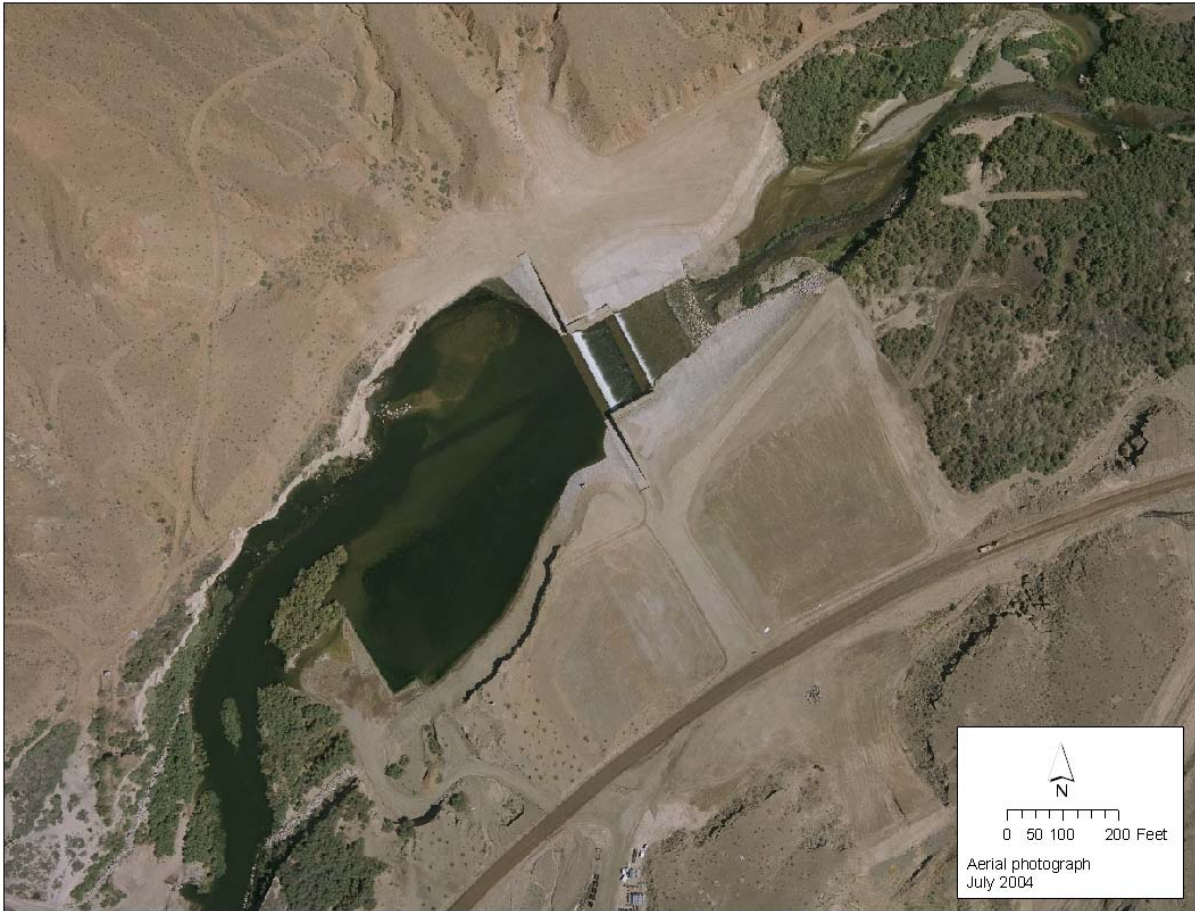
Figure 2: Completed Rainbow Gardens weir.
