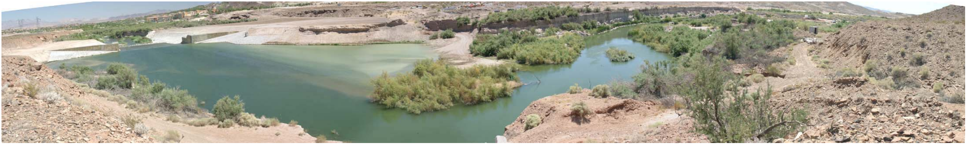
August 2004 image of the Rainbow Gardens weir location (after construction)
