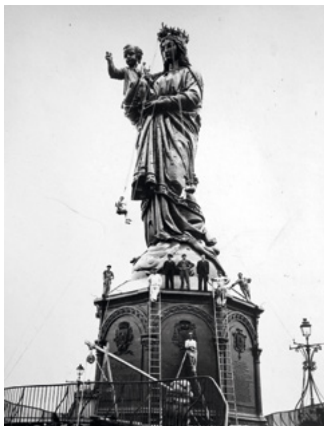
Restoration work on the Notre-Dame de France statue, 1937
