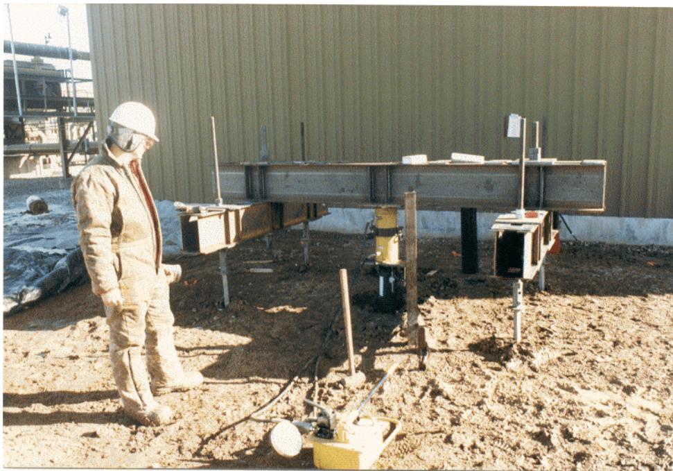
Figure 15.1: Full Scale Compression Load Test
