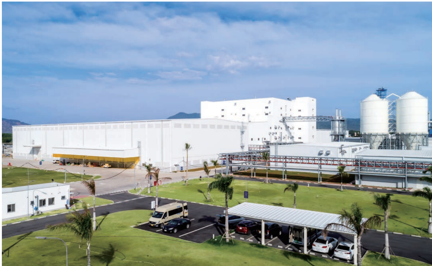
Iguacu Vietnam Soluble Coffee Manufacturing Plant (Vietnam)
