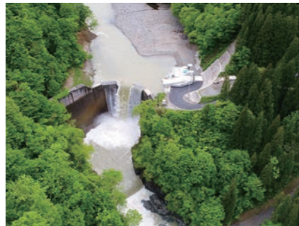
Kamiketto Hydro Power Plant (Tsunan-machi, Nakaonuma-gun, Niigata)
