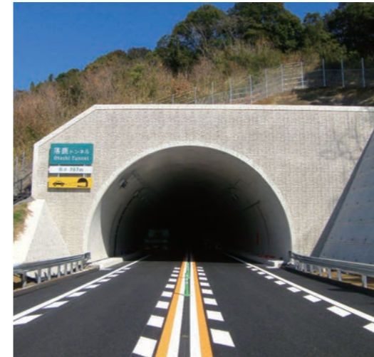
Higashi-Kyushu Expressway Otoshi Tunnel (Hyuga-shi, Miyazaki)
