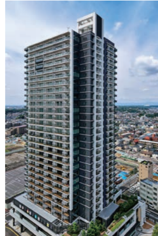
Redevelopment of a category 1 urban district in the north block near the West Exit of Tokorozawa Station (Tokorozawa-shi, Saitama)
