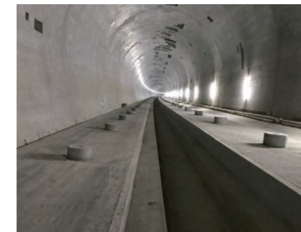
Kakibara Tunnel (Awarashi, Fukuji)
