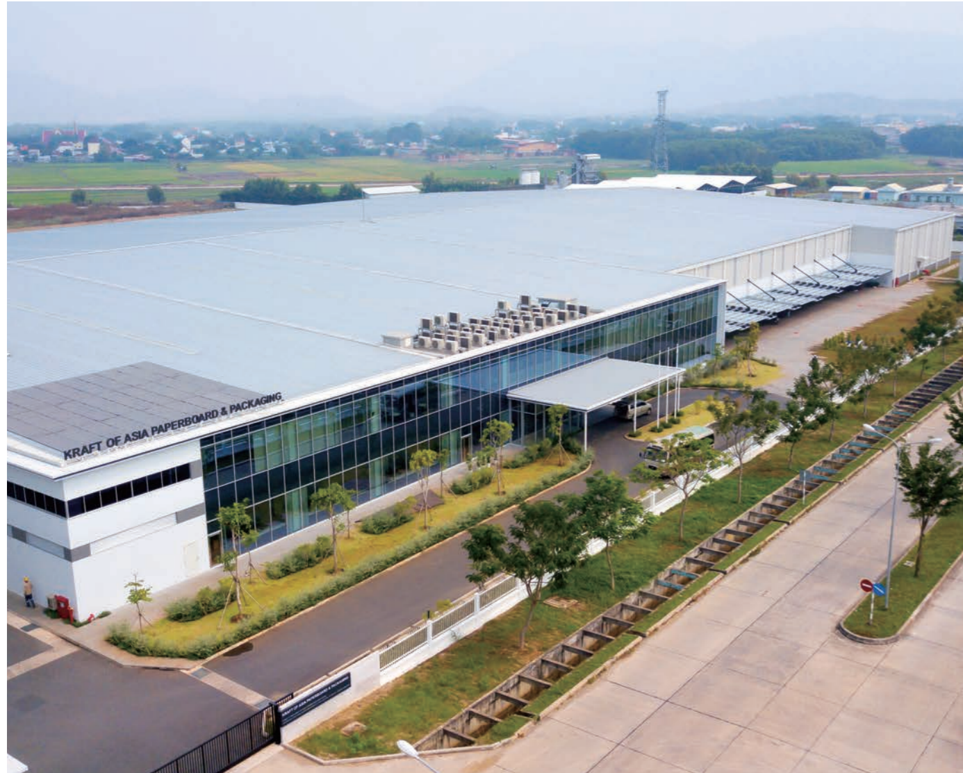
Liner Mill Project in Ba Ria-Vung Tau Province (Vietnam)
