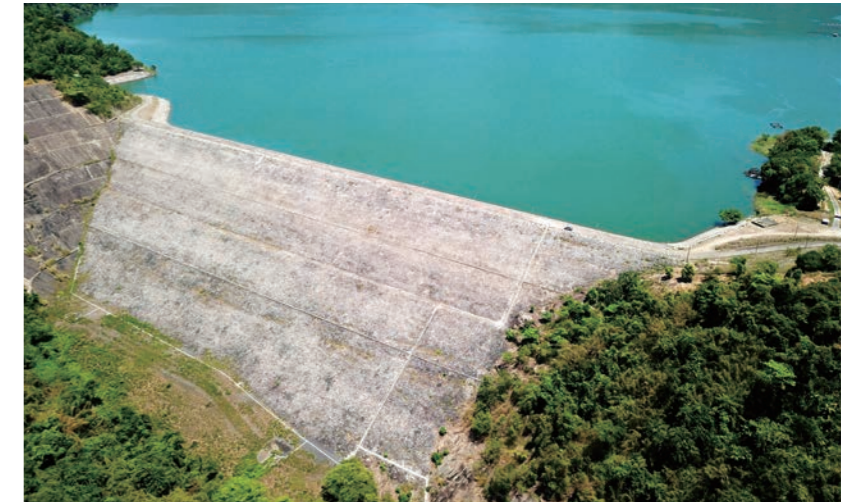
Da Mi Hydro Power Plant (Vietnam)
