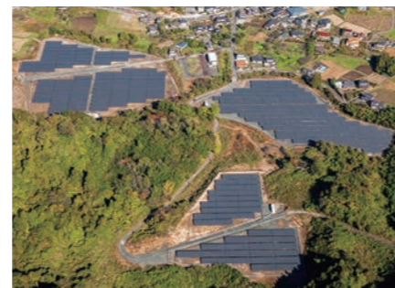
Kitaibaraki Solar Power Plant (Kitaibaraki-shi, Ibaraki)
