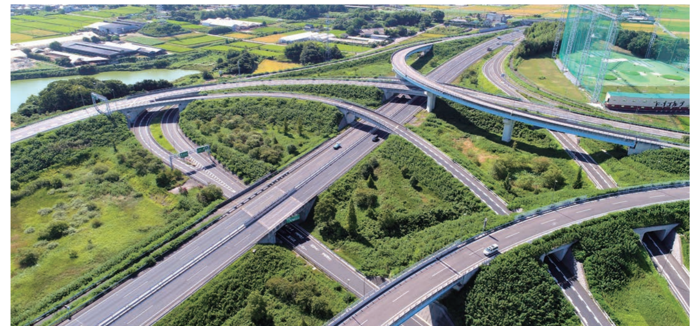
Aichi Prefectural Toll Road (Aichi)
