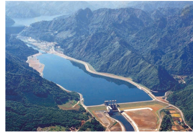
Tadami Hydro Power Plant (Tadami-machi, Minamiaizu-gun, Fukushima)
