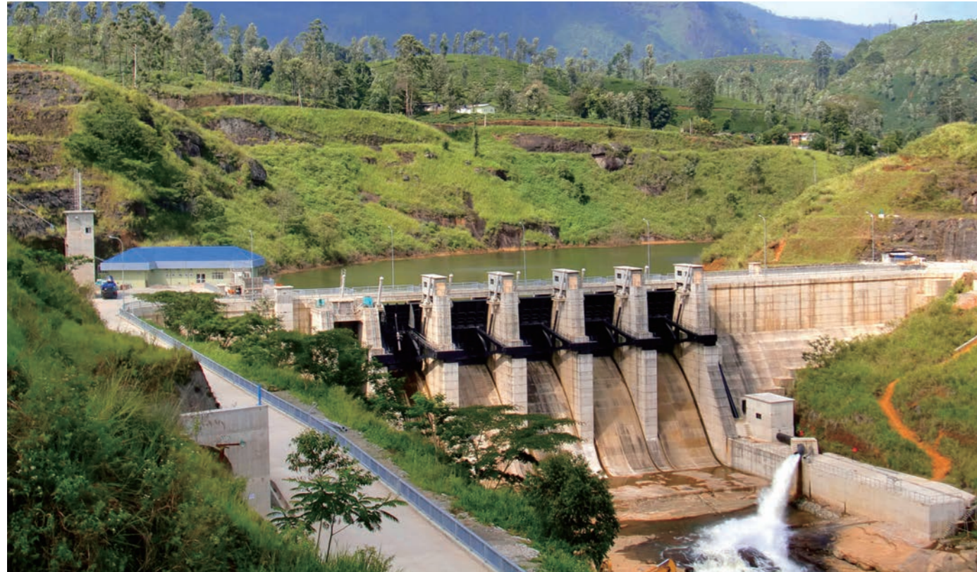
Upper Kotmale Hydro Power Plant (Sri Lanka)
