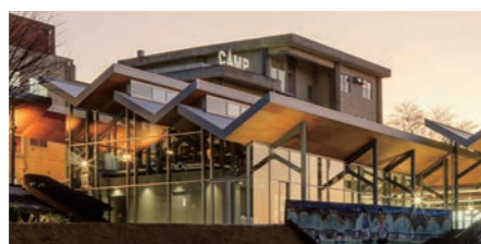
ICI Camp This facility is equipped with various seminar rooms and meeting rooms, has accommodation with capacity for approximately 200 people and a sophisticated dining room, and is optimal for training, research and development.
