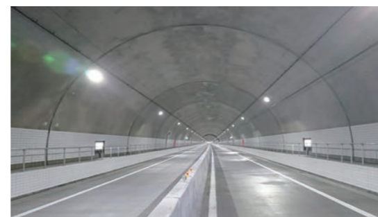
National Route 45 Shinkuwadai Tunnel (Ofunato-shi, Iwate)
