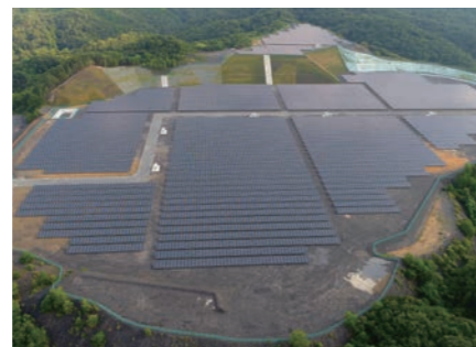
Mine Solar Power Plant (Mine-shi, Yamaguchi)
