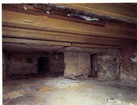
Originally, the distance to the ceiling in the cellar room was only 1.8 metres, but after excavation the distance is now 2.5 metres. The two photographs show the reception area before and after the extensive restoration.
