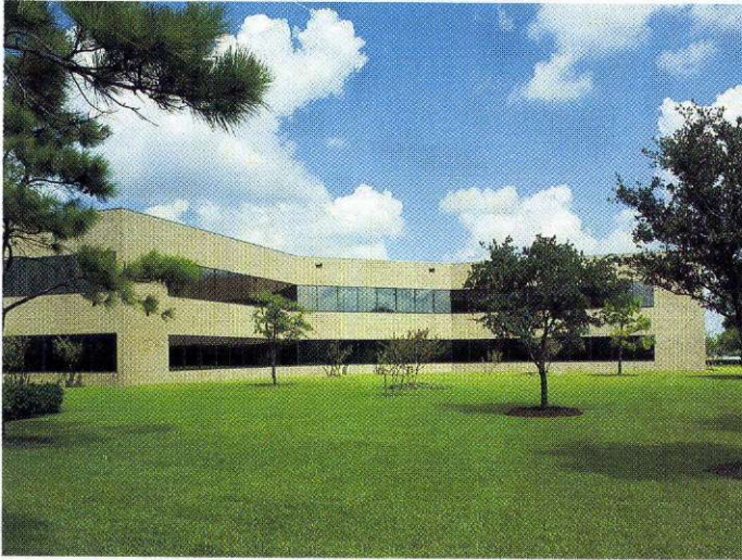
The new Houston headquarters for Maersk Inc., APMC, Moller Supply, Maersk Drilling, and Maersk Energy.
