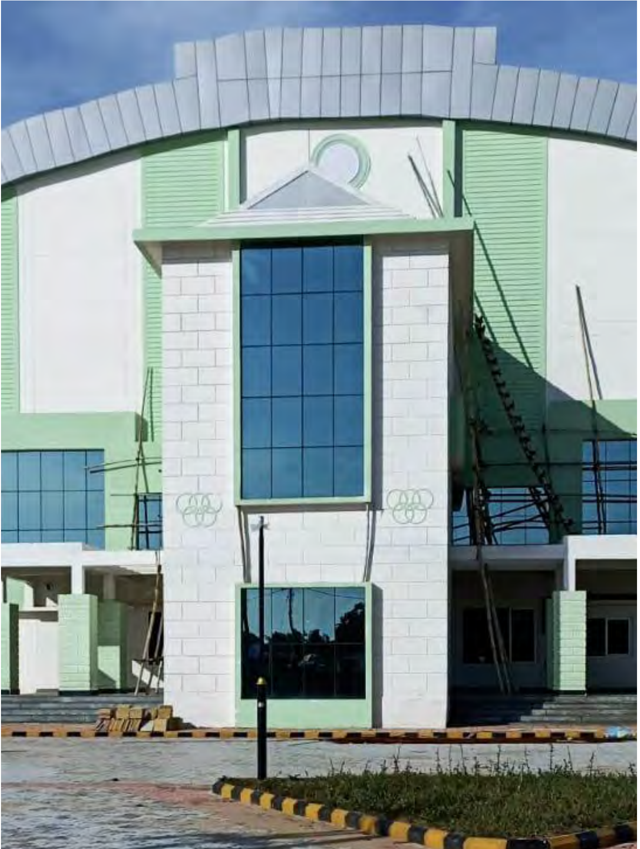
Multipurpose indoor stadium, Jajpur
