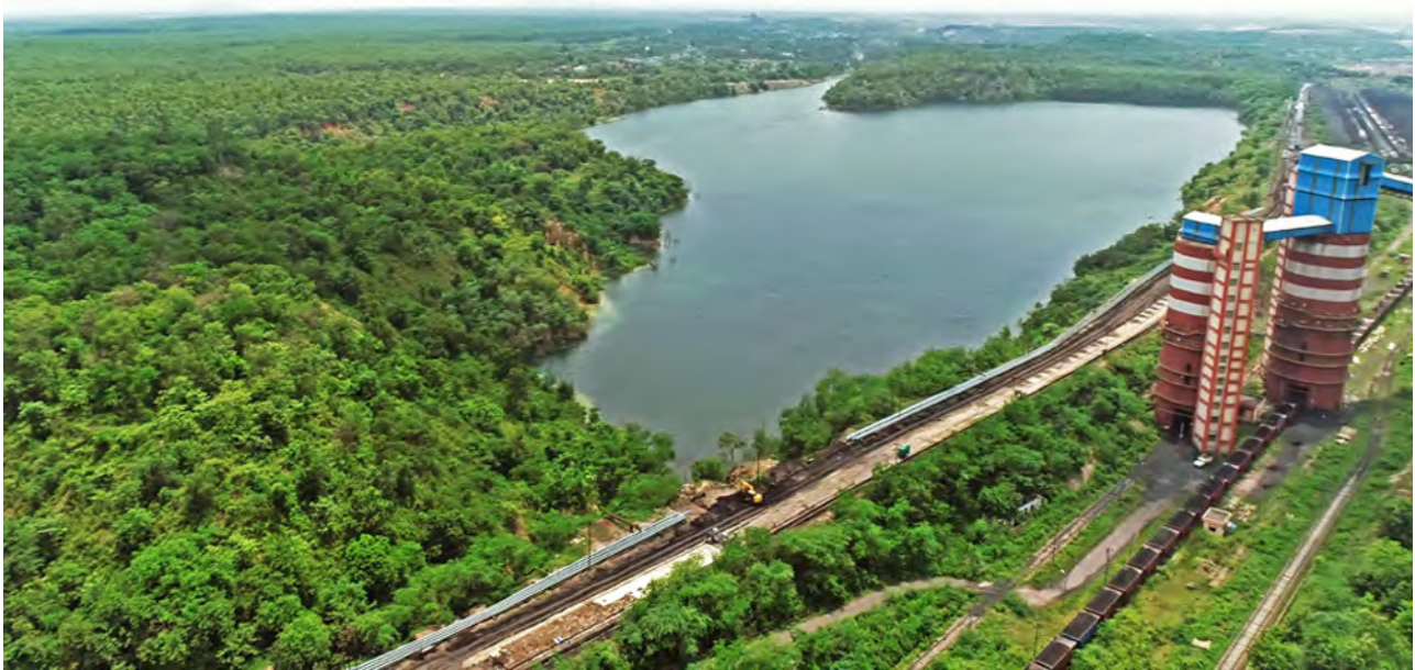
Arial View of Bharatpur FMP Project
