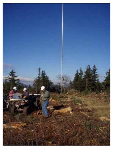
Figure B-3b: A tubular structure with guys and mulched guy corridor
