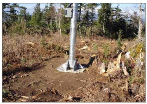
Figure B-3a: Base plate of a tubular met tower
