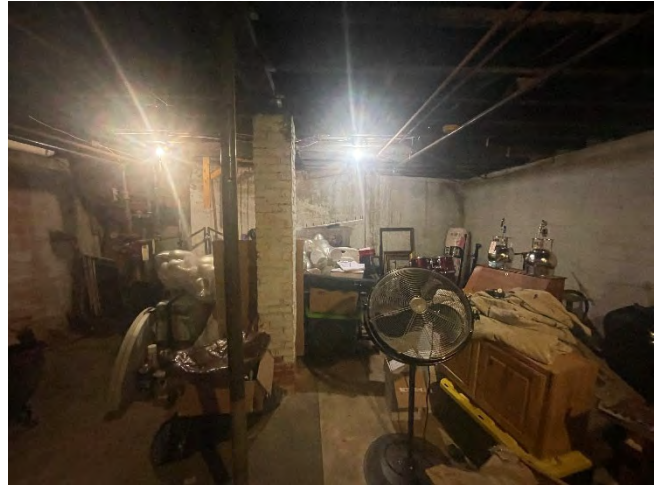
Description: Photo Studio Basement.
