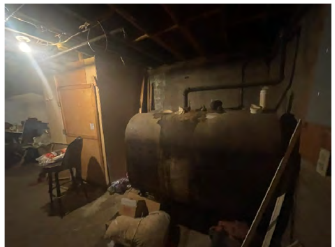
Description: Photo Studio Basement, AST location.
