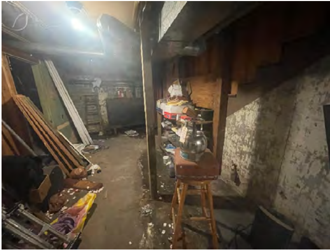
Description: Pawn Shop Basement (55 State St.), Sample AS-2 location
