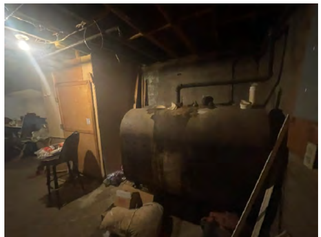
Description: Photo Studio Basement, AST location.
