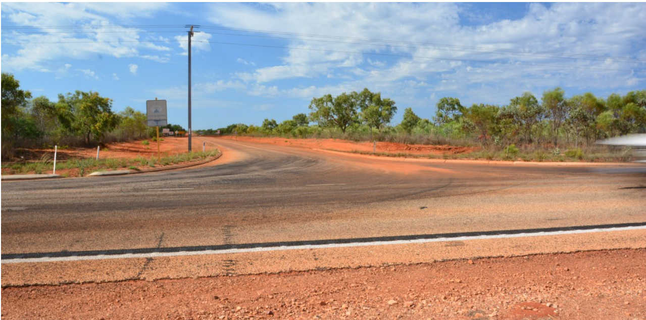
Plate 1: Existing Intersection of the Broome-Cape Leveque Road with Broome Highway
