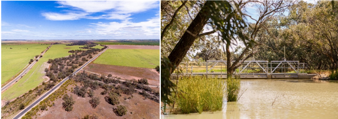
Figure 59: Yarriambiack Creek and Beulah Weir Pool.
