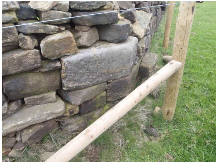
masoned quoins as park wall turns NE immediately N of the old quarry at Swallow Head
