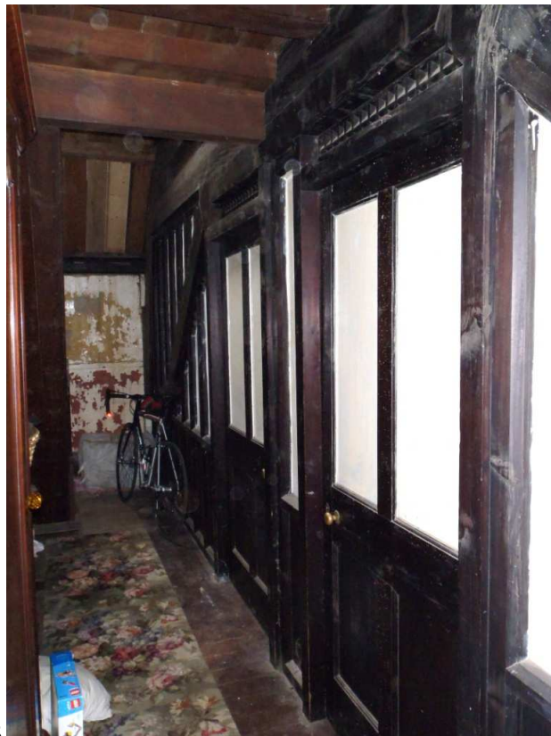
original asbestos panels
