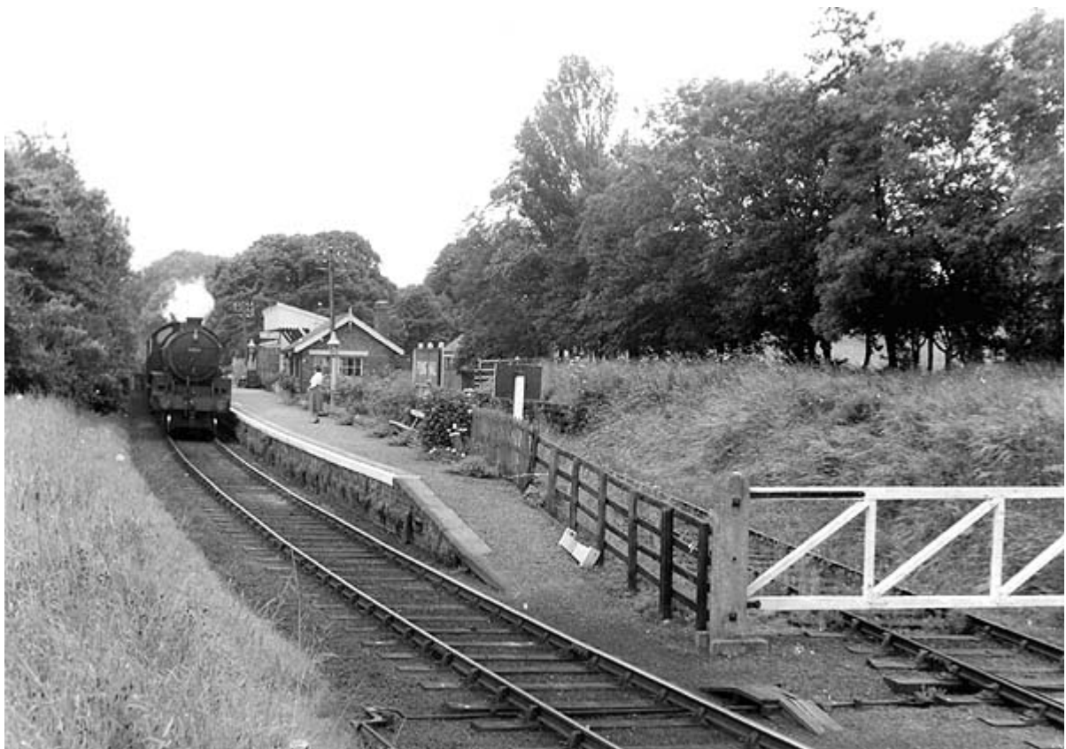
Fyling hall station looking south in the 1950's
