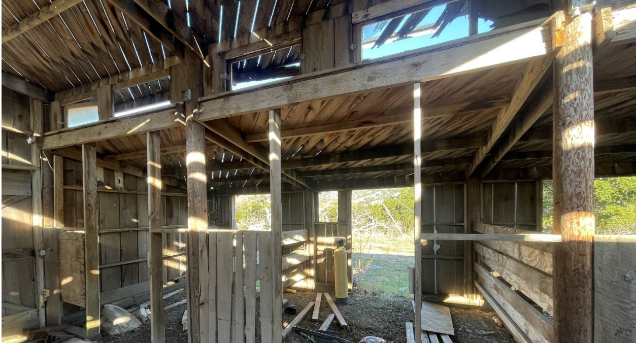
Photo 6. Interior view of the dilapidated barn in the Study Area. Large openings and gaps present on the roof and sides of the structure. Photo taken on November 28, 2023.
