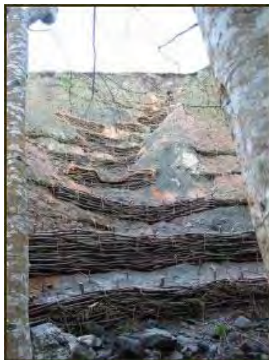
Close up of willow walls shortly after planting.
