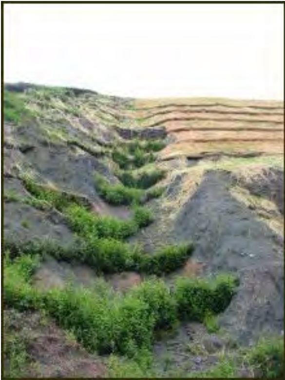
Before, during, and after photos of a slide repair at Olema Creek using willow walls, straw wattles, fabric, and seed.
