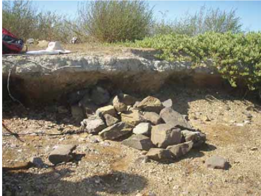
Photo 9. Rock micro-groin, as constructed on 9/15/2009
