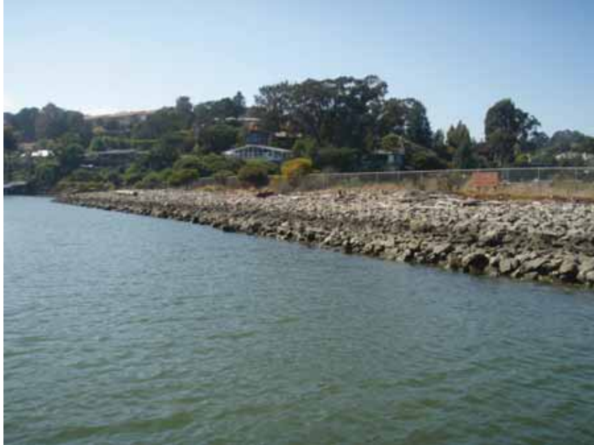
Photo 5. Rip-rap revetment along southern island shore (photo by Stuart Siegel, 9/12/2008)
