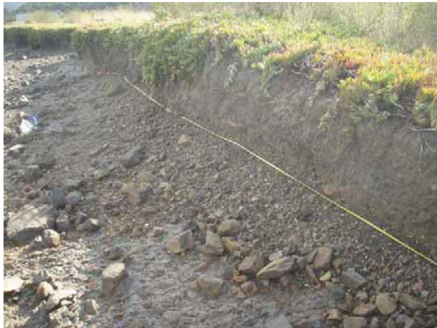
Photo 5. Feature 3, gravel toe berm
