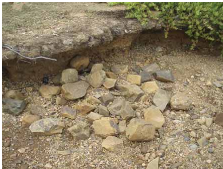
Photo 10. Rock micro-groin after the storm
