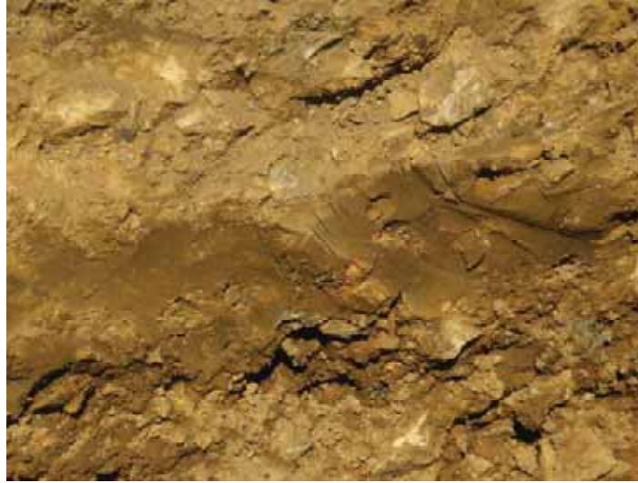
Photo 10. Trench 3, soil layer 2 (stiff clay) between layers 1 and 3
